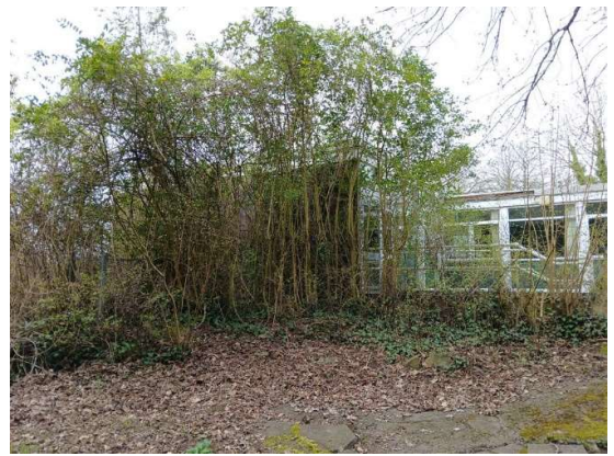
East Elevation (South end)
