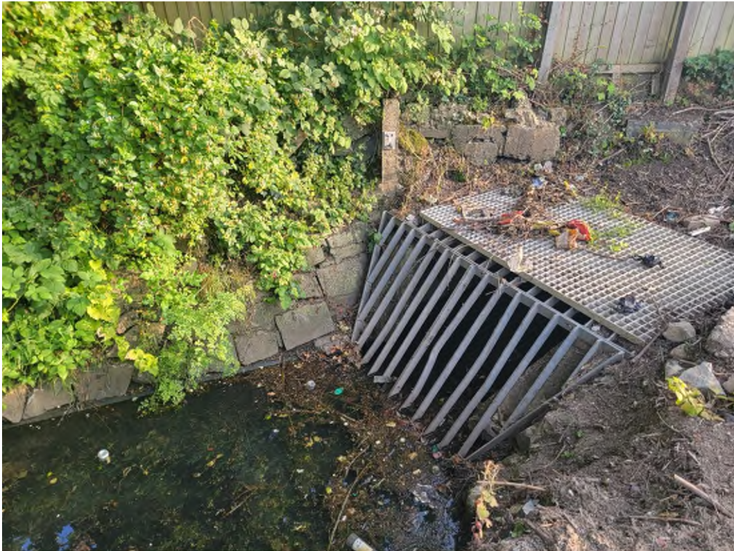
Figure 7 – Watercourse headwall into culverted section.
