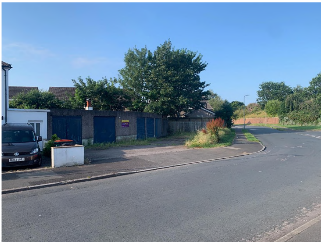
Figure 4 – The site from Thompson Avenue
