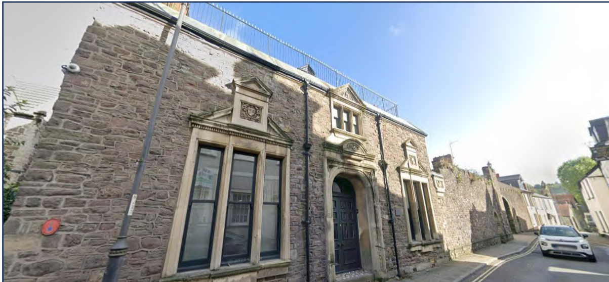
Traditional Victorian civic architecture with symmetrical stone façades, ornate pediments, arched entrances, sash windows, and classical detailing conveying historic authority.
