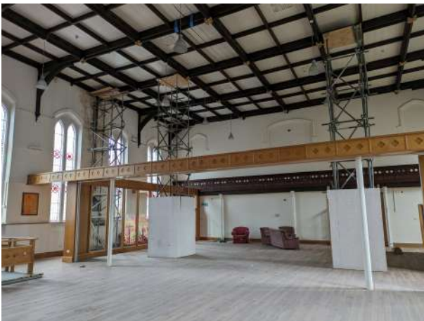
4. The interior space with modern screen and propping.
