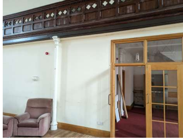
8. Cast iron columns supporting former gallery and entrance to offices and WCs
