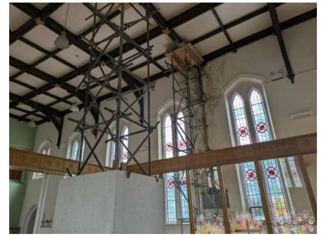
9. Scaffold propping of main ceiling
