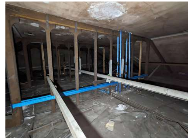
6. Queen post trusses with additional strapping
