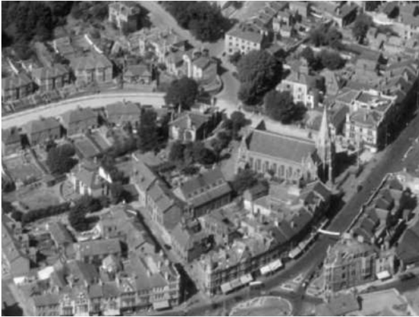
1. Aerial photograph WAW010619 WALES (1947)
