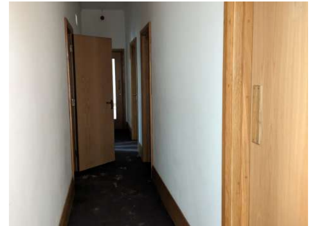
12. Offices in west end, not of merit
