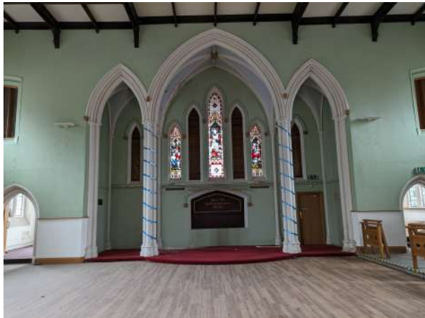
10. The chancel /apse windows
