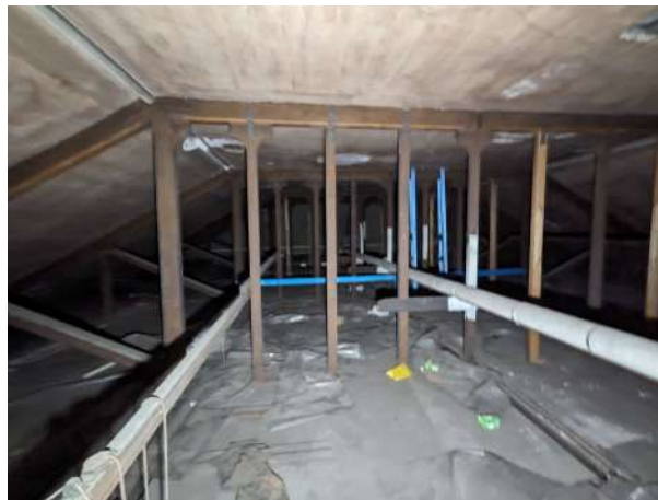
5. View of roof space and Queen post trusses
