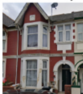
Front of Building
