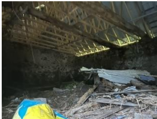
Figure 24 Trussed roof to right hand room.
