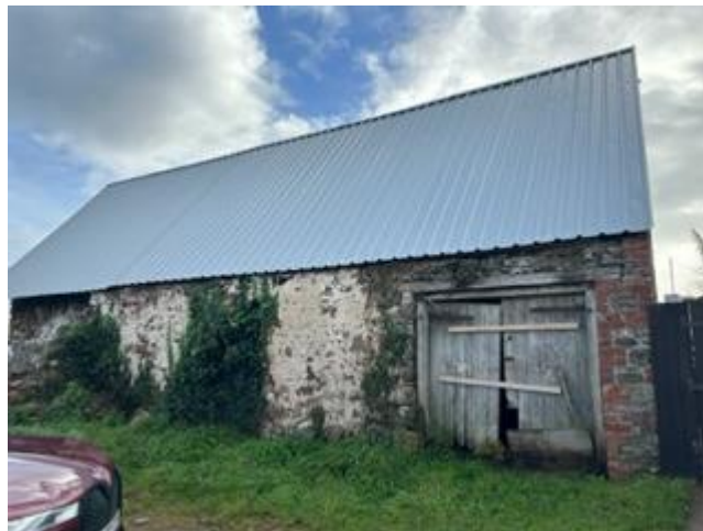
Figure 2 Front (Coc Y North Road) elevation 2 of 5
