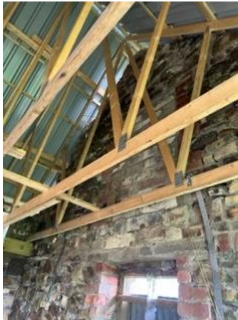
Figure 11 Internal trussed roof
