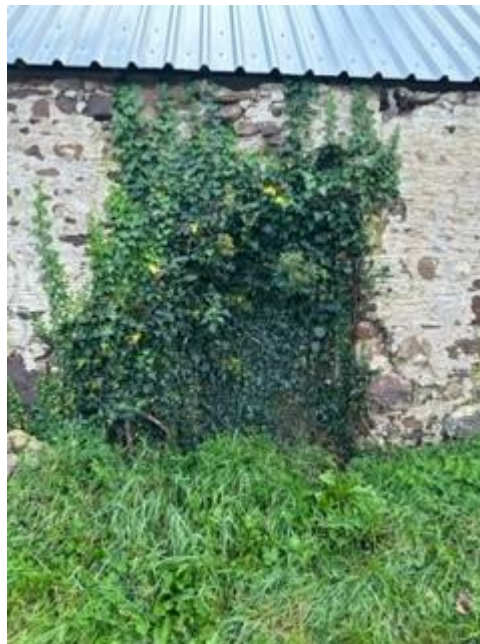
Figure 4 Front (Coc Y North Road) elevation 4 of 5
