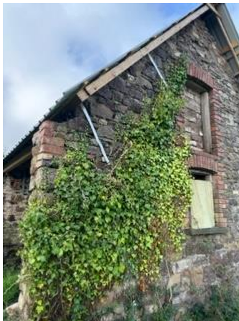
Figure 8 Left hand side of gable end.
