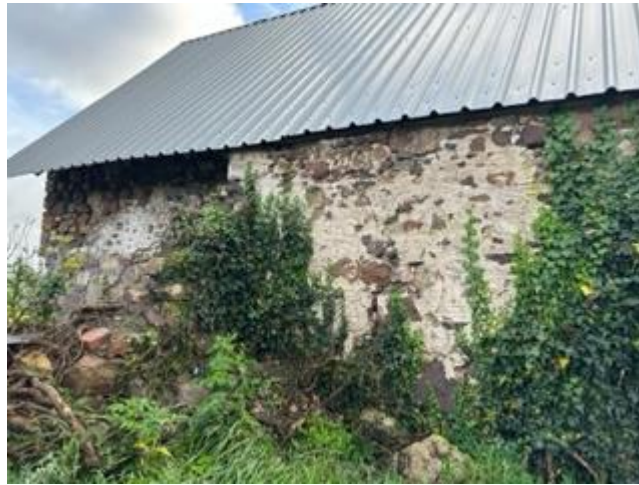
Figure 5 Front (Coc Y North Road) elevation 5 of 5
