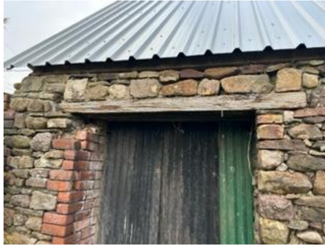
Figure 23 Lintel to structural opening.
