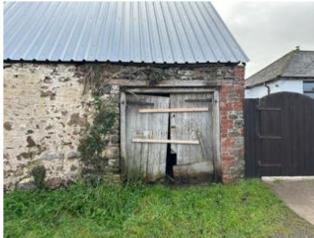
Figure 1 Front (Coc Y North Road) elevation 1 of 5
