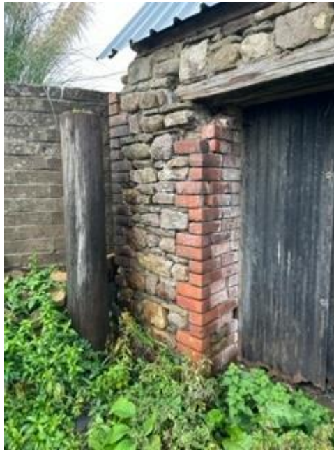
Figure 21 Brickwork reveals to structural opening.
