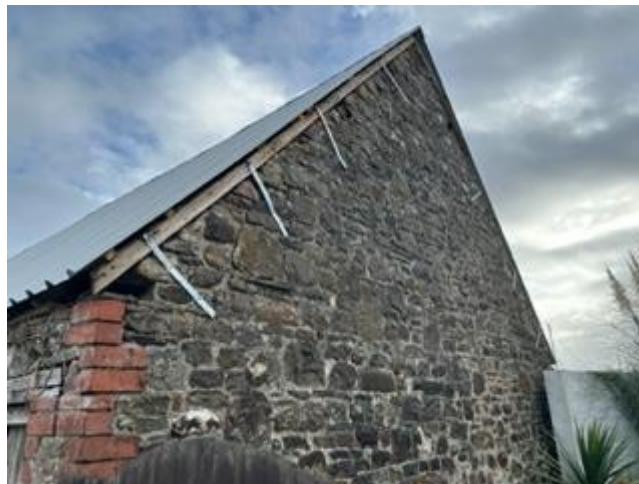
Figure 26 Right hand gable.
