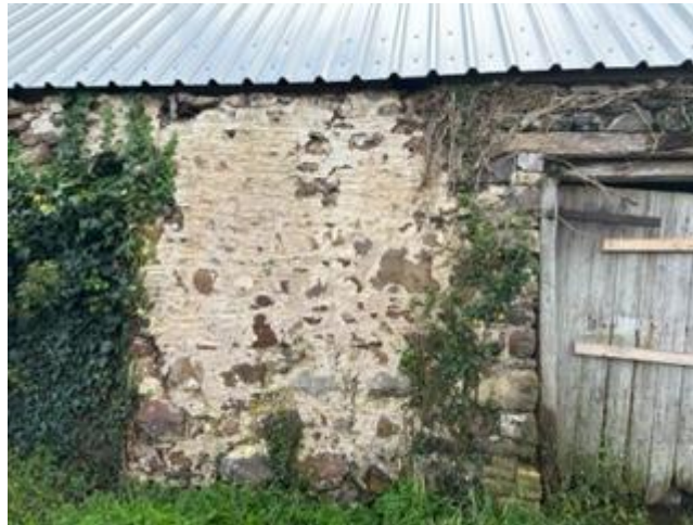
Figure 3 Front (Coc Y North Road) elevation 3 of 5
