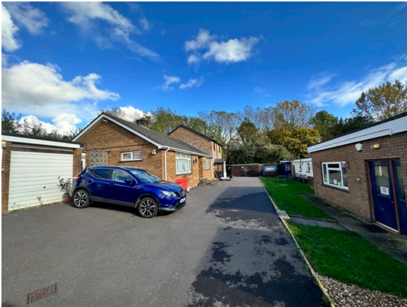
Photo B : View of the existing bungalow facing back towards the main entrance.
