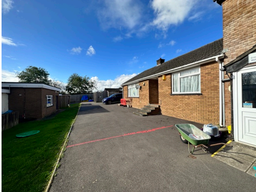
Photo A : Front elevation of the existing bungalow
