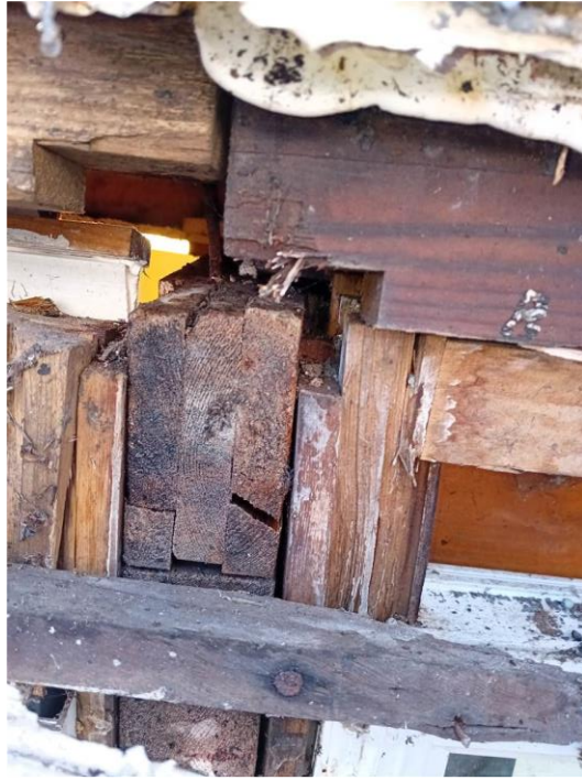
Above: external opening-up works of typical beam-post connection, revealing extent of movement
