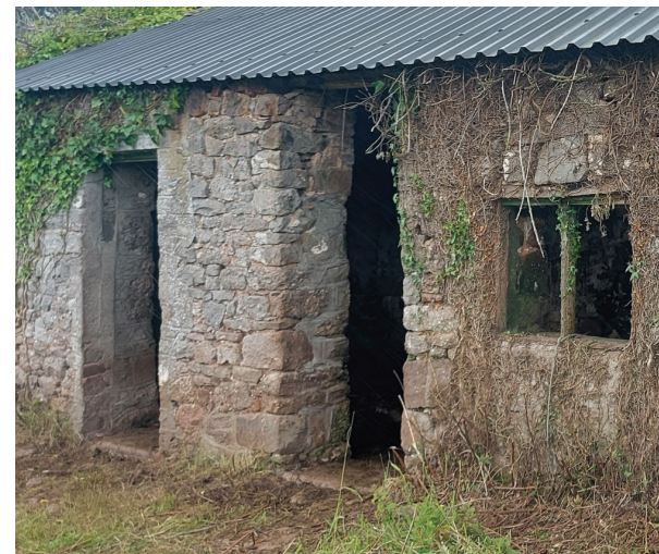
Existing external openings
