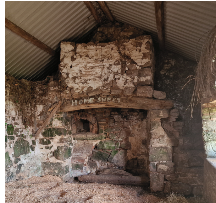
Existing inglenook fireplace with partial staircase to the side
