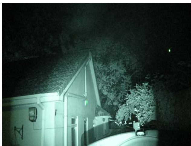
Photo 2. The northwestern and northeastern elevations of the main building of the day centre at the darkest point of the survey on the 14 th May 2025 from NVA location 2.
