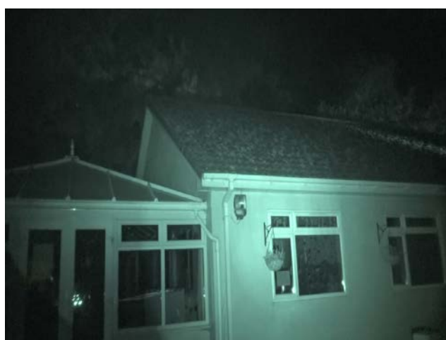
Photo 4. The northeastern and southeastern elevations of the main building of the day centre at the darkest point of the survey on the 4 th June 2025 from NVA location 1.
