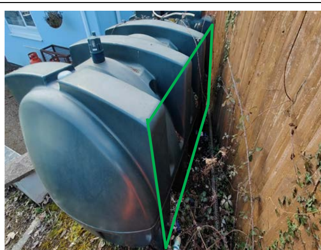
Photo 18. The northwestern elevation of the fuel storage container (green).
