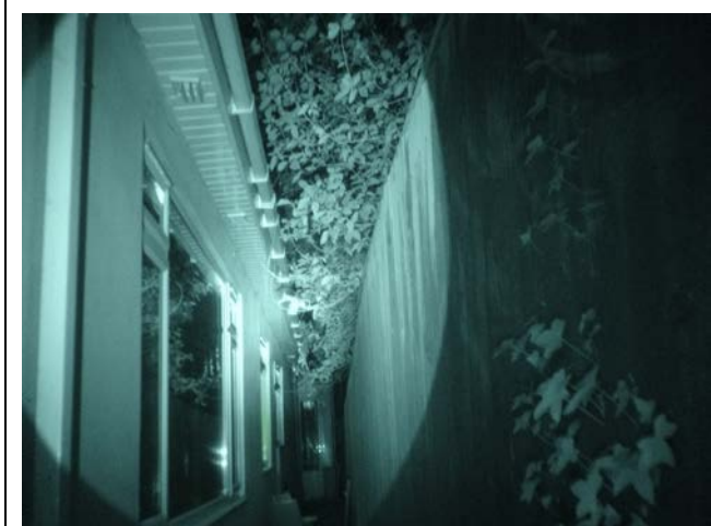
Photo 3. The southwestern elevation of the main building of the day centre at the darkest point of the survey on the 14 th May 2025 from NVA location 3.
