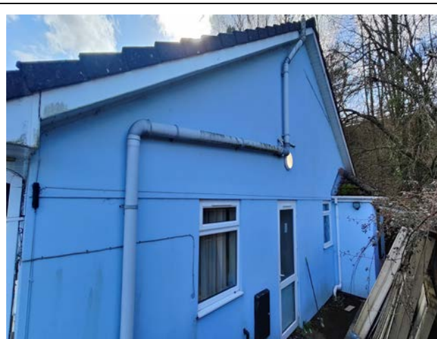
Photo 12. The northwestern elevation of the day centre main building.
