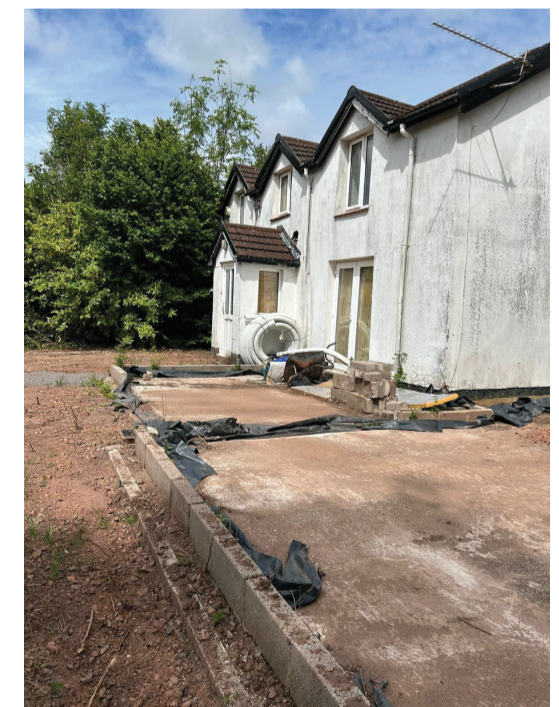
PHOTOS OF EXTENSION
