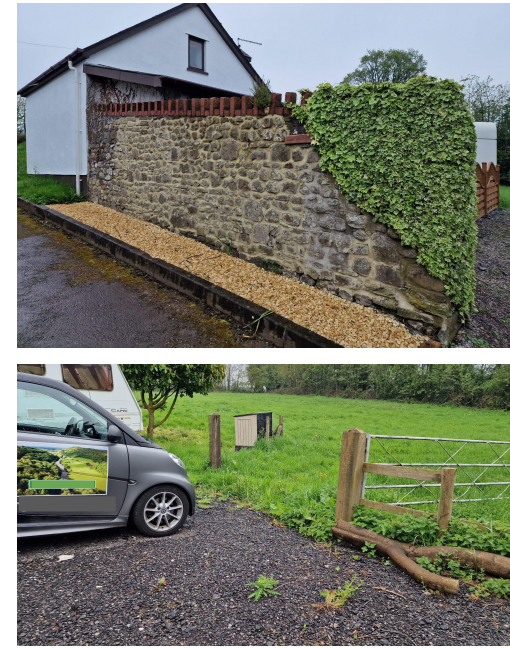
Figure 9 - Existing access and parking
