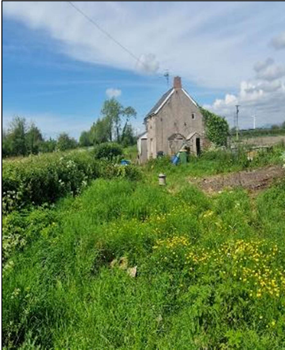
Plate 3: Summerleaze Cottage and the eastern end of the development site
