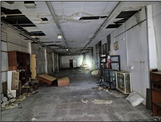
Figure 11 – (W) Ground Floor Interior of Survey Building, Looking (E)
