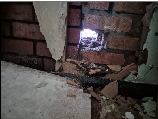
Figure 5 – Hole visible in Figure 4 from Interior of Building. Presence of Cobwebs across Span of Gap Suggests the Potential Access Point is not being Utilised by Bats
