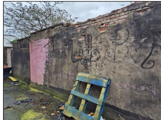
Figure 10 – Damaged Masonry / Render Covering Brickwork on (S) Wall of Flat Roof of Building, Offering Potential Limited Roosting Opportunity for Crevice-Dwelling Bats
