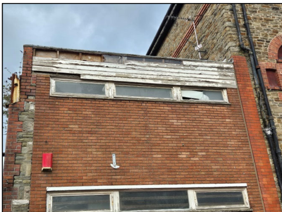
Figure 6 – (E) Wall of Survey Building Looking (W). Damaged Windows and Fascia / Cladding Boards visible, Enable the Potential Access/Egress for Bats to the Building Interior
