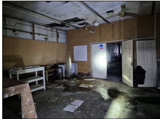
Figure 14 – Damage to Underside of Flat Roof as a result of Water Ingress above Stairwell at Far (E) Section of Building Interior.
