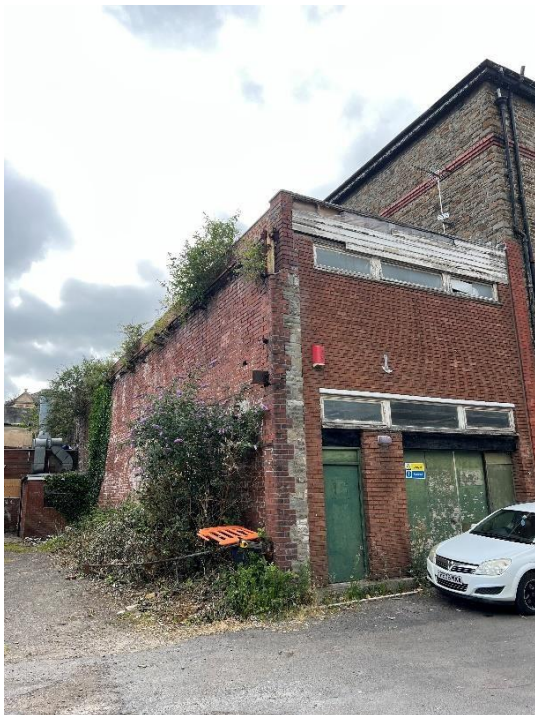
Fig 9 Rear view of existing building
