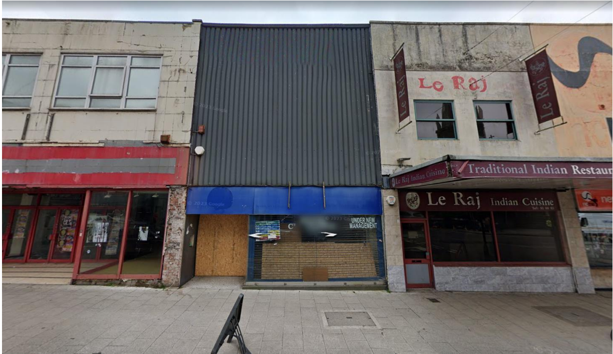
Fig 5 Front view of site existing
