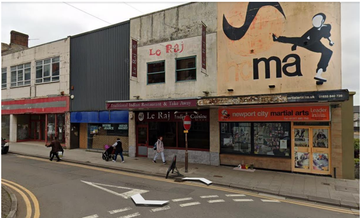
Fig 6 View of 84-85 commercial street (LeRaj Restaurant Vacant and Derelict)
