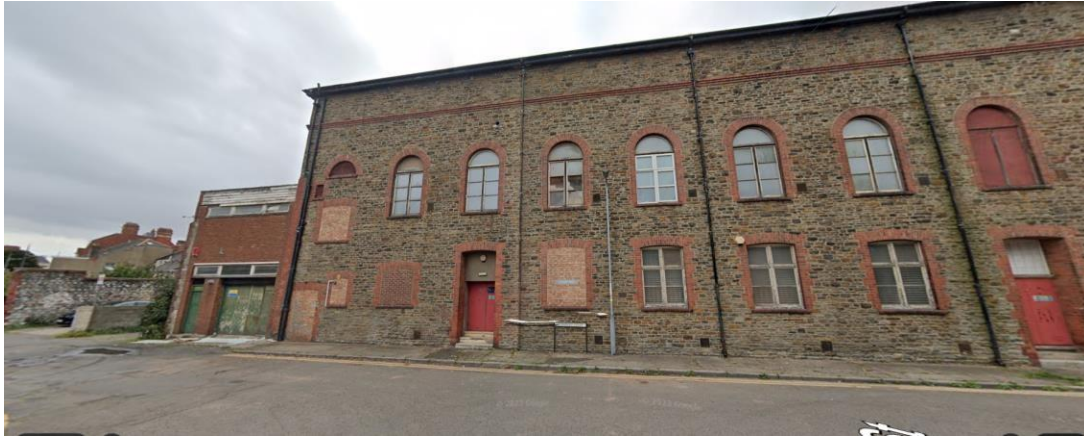
Fig 8 View of adjacent building to north on rear
