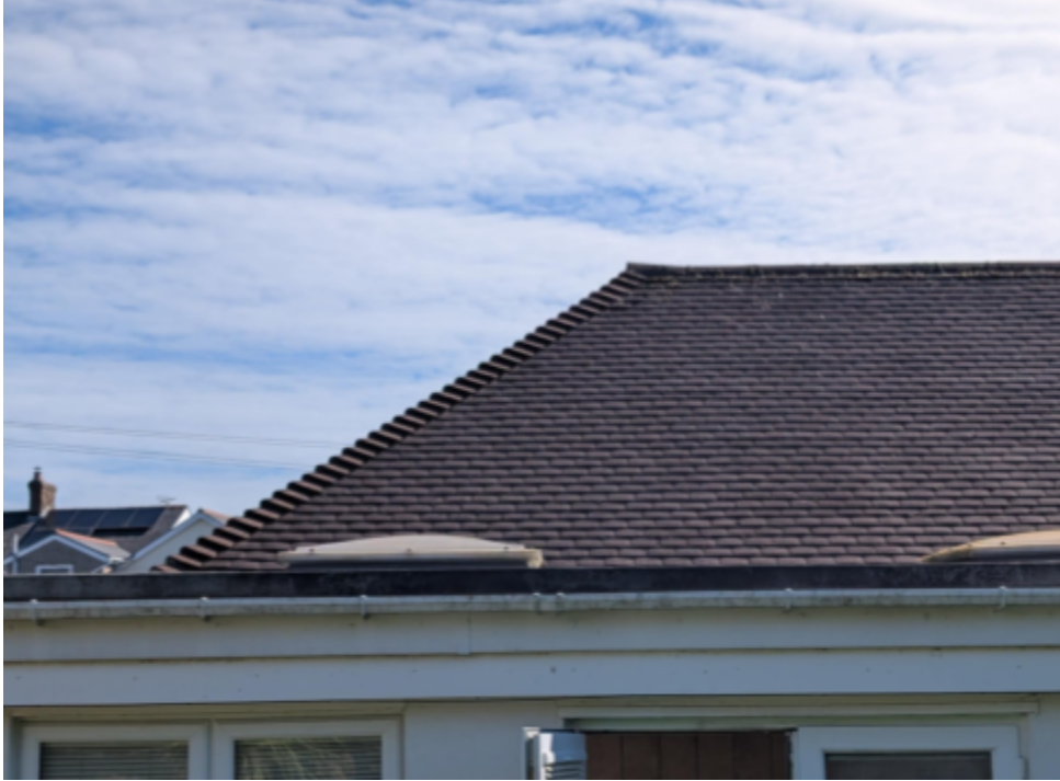
Plate 1- example of tightly fitting tiles and flat roof
