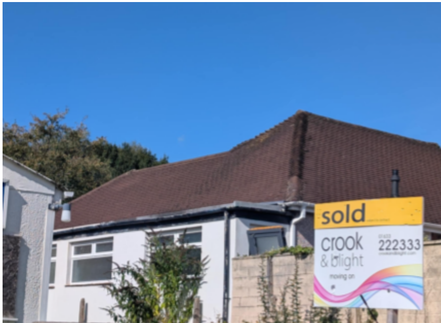
Plate 4- sealed area where a chimney has been removed
