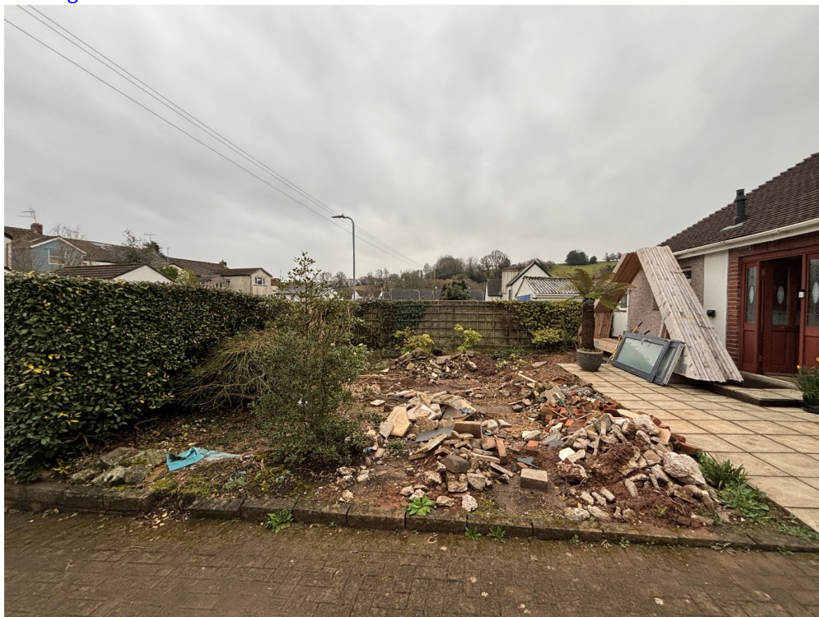
Front garden – hard surfaces in process of being grubbed up
