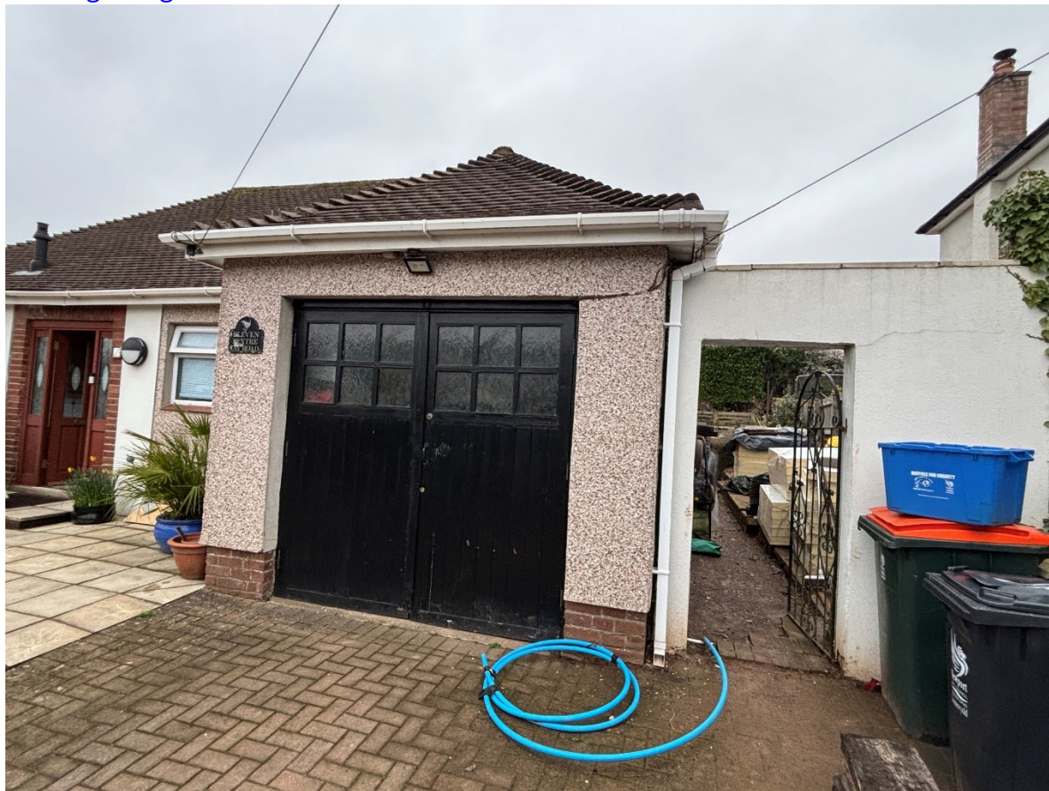
Existing front elevation – hard surfaces to be removed
