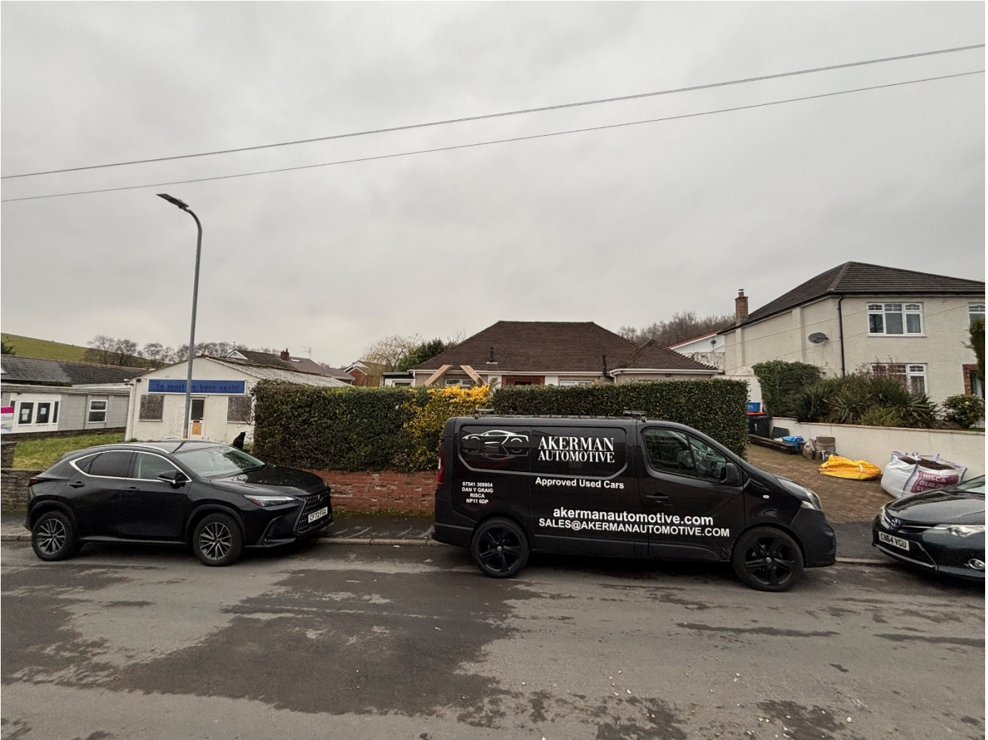
Street Elevation – r/h section of wall and hedgerow to be removed to improve site access (3.5m length)
