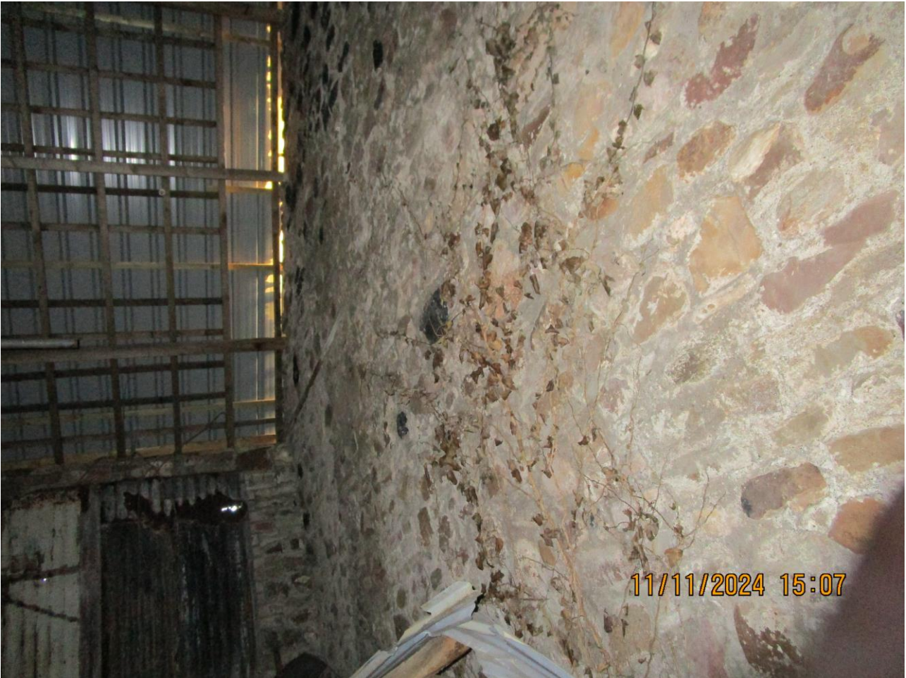
Purlins and rafters – right-hand side
