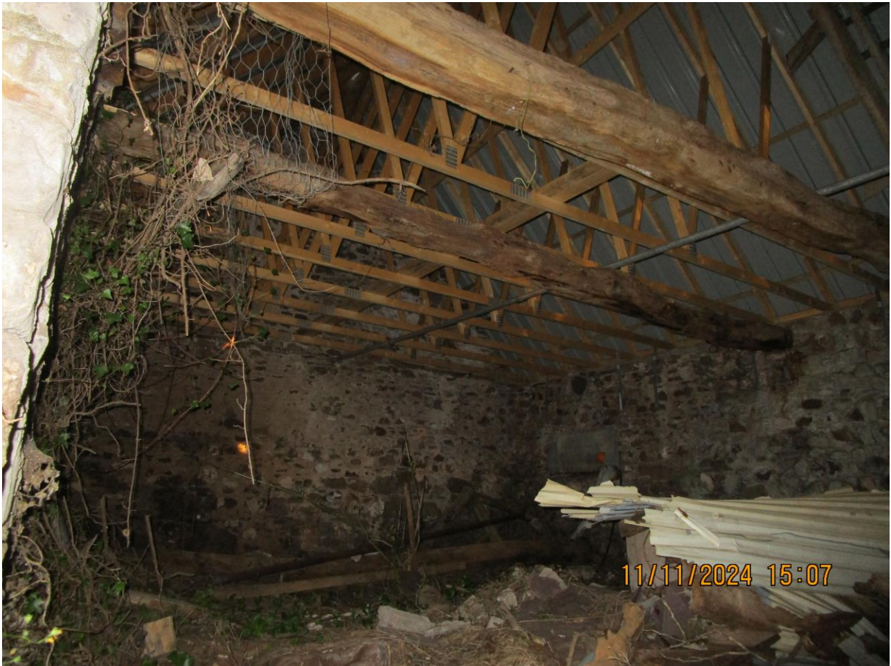
Timber trusses – left-hand side
