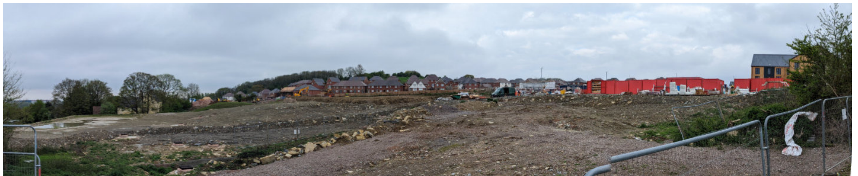
Image of construction site from Milton Hill road.
