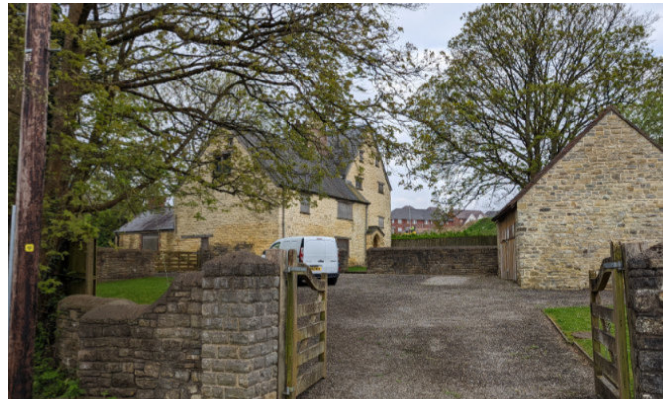
View 4 - View through gate of Great Milton House
