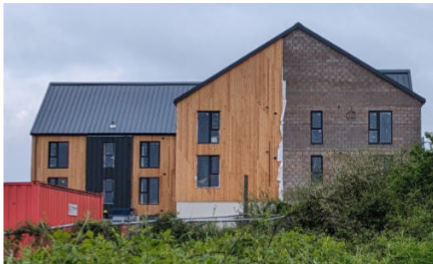
New block of flats Great Milton Park - Timber Cladding
