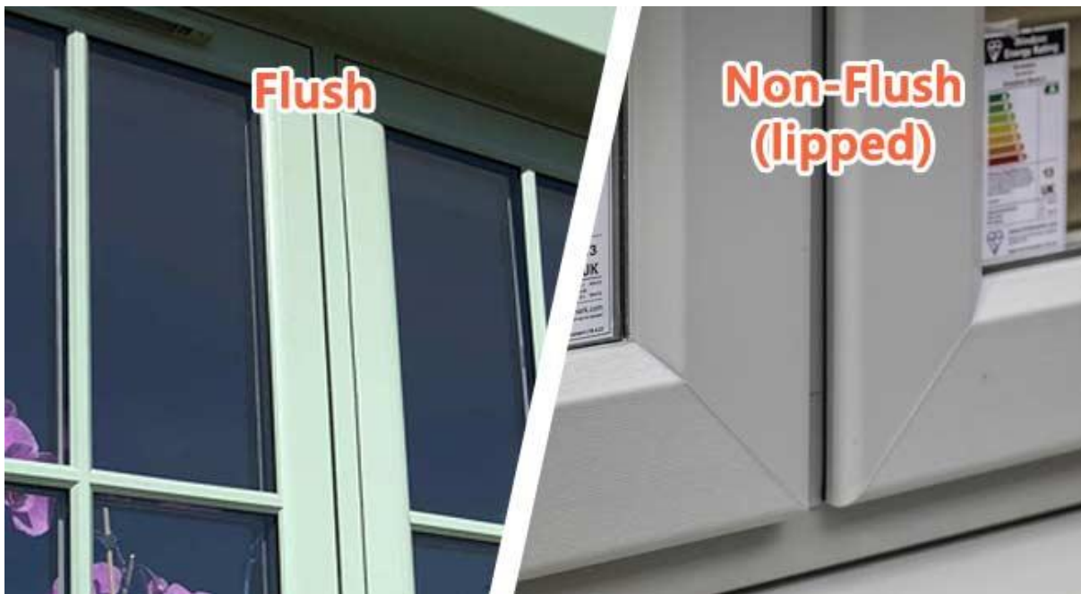
Images indicate the difference between a non-flush (lipped) window frame, widely used in modern construction, and a flush fit window frame resembling the look of traditional timber casement windows.
