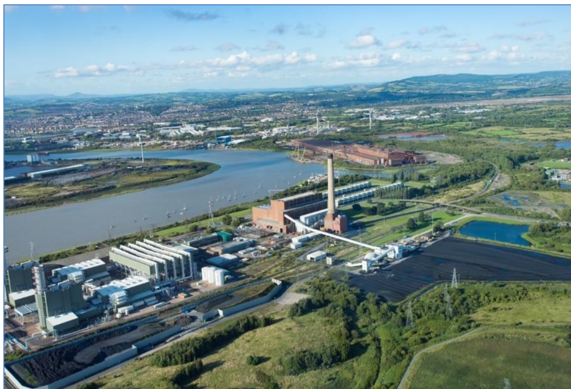
Figure 4 Uskmouth Power Station and former coal stockyard
