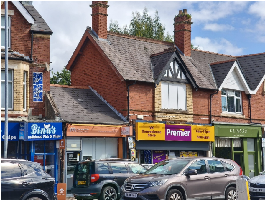
Picture 1: View of front elevation
