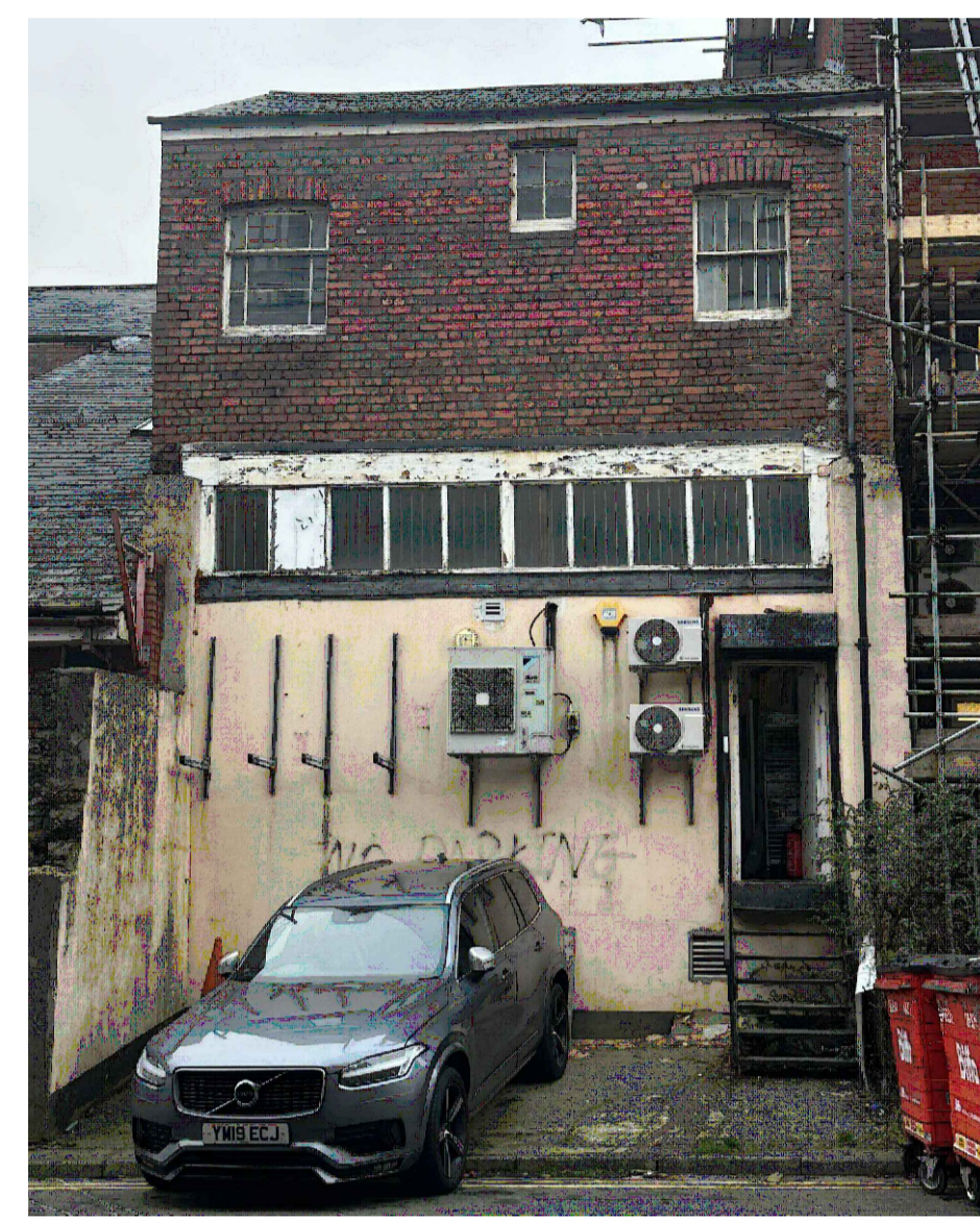
Rear view - East - Existing
