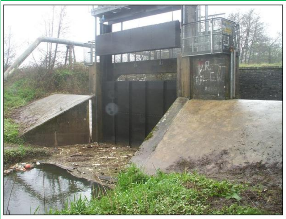
Figure 4 - Gwastad Mawr Sluice
