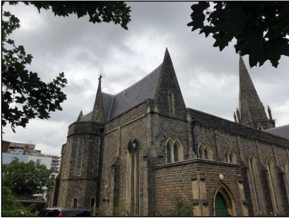
Photo 1 – West and Southern Elevations
