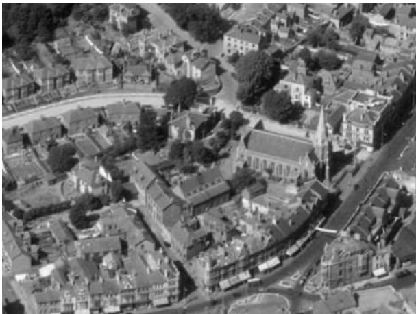
11. Aerial photograph WAW010619 WALES (1947)
