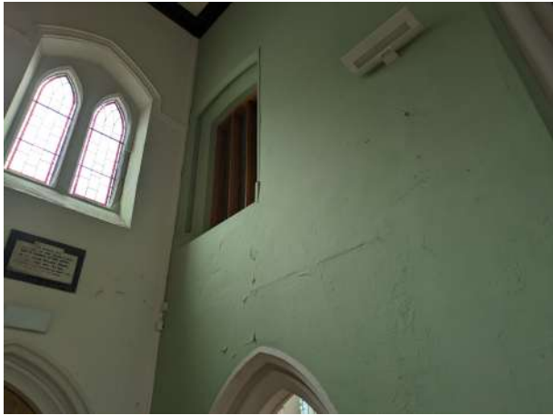
5. Gallery door in east end
