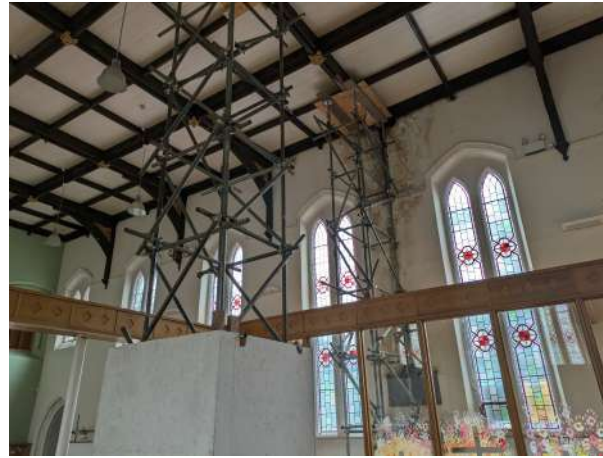
9. Scaffold propping of main ceiling
