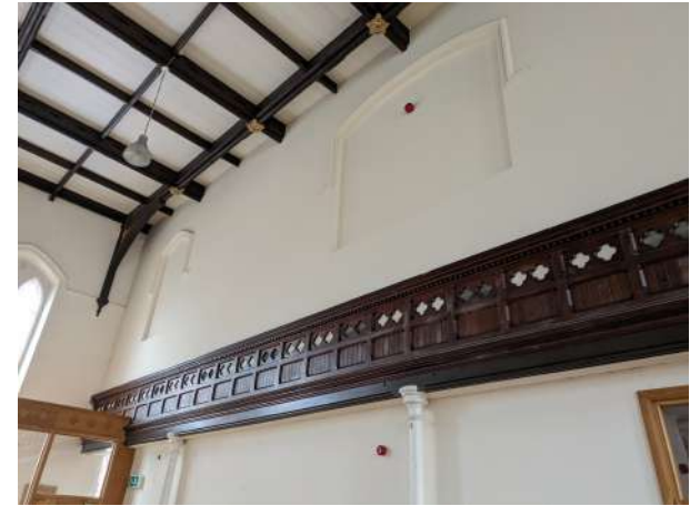
7. Wooden frontal piece to removed gallery in west end
