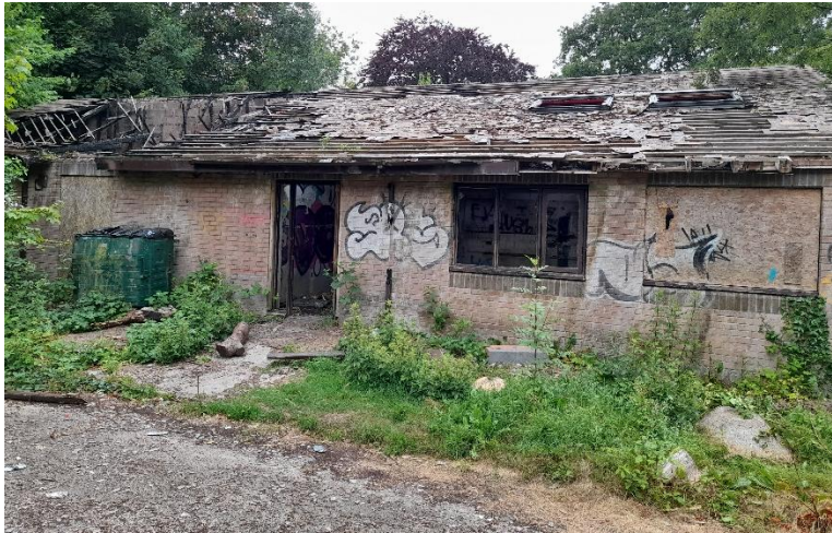
Existing Building on site (Previously Kensington Court Day Centre)
