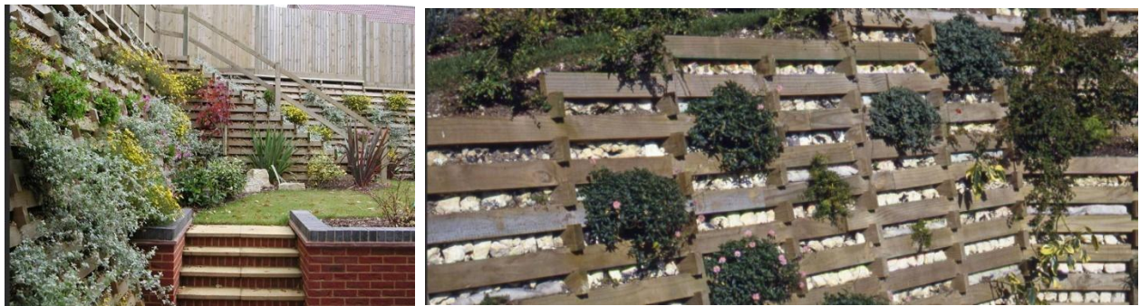
Examples of Crib Lock Walling with Planting
