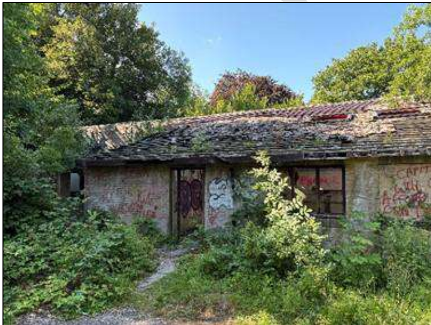
Plate 3 – Main building located at the site centre.
