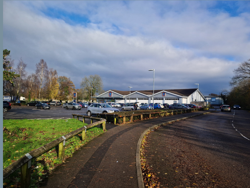
Figure 10 - Supermarket at Nash Road
