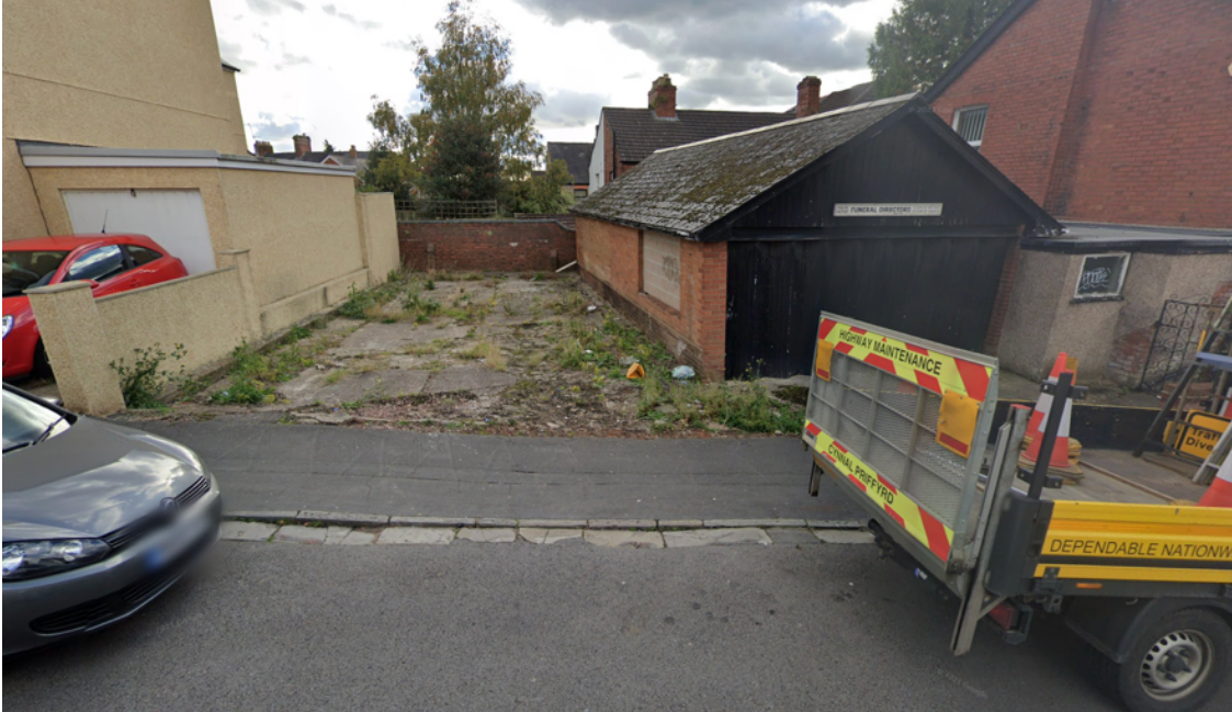
Figure 2 Existing Garage & Yard Area
