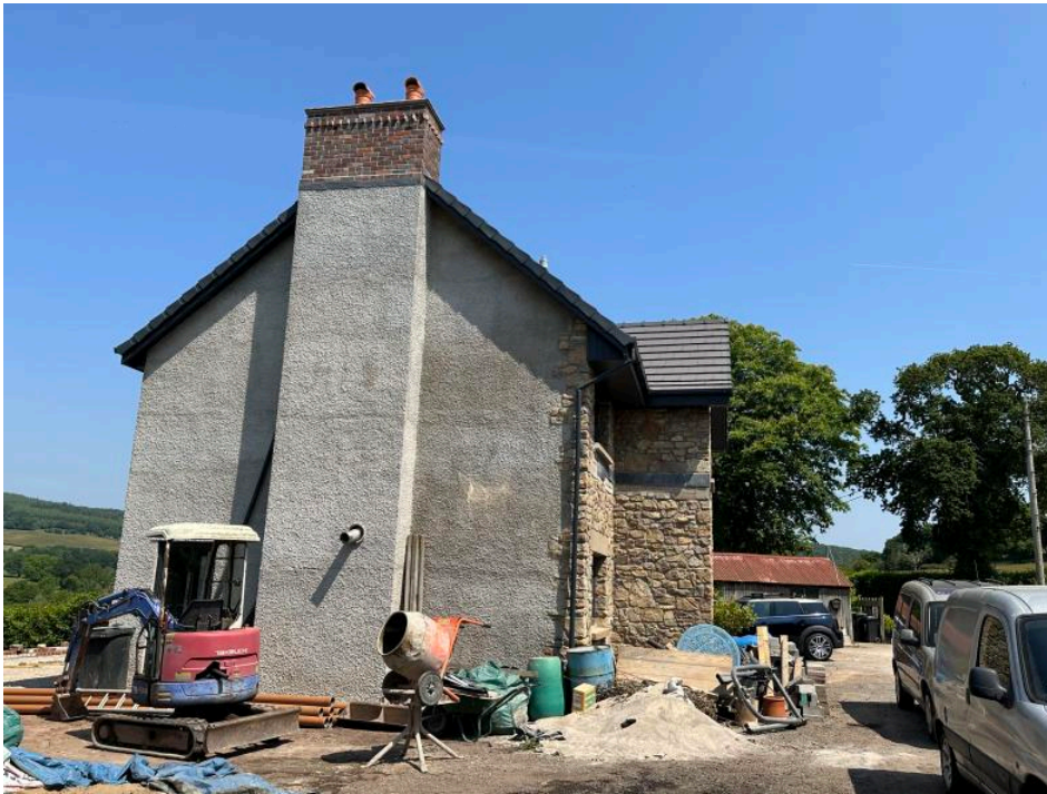
Fig 4: Partially built house and area to south side.
