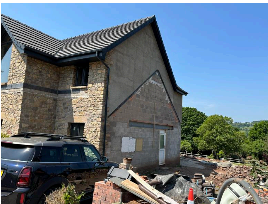
Fig 3: Partially built house and area to north side.
