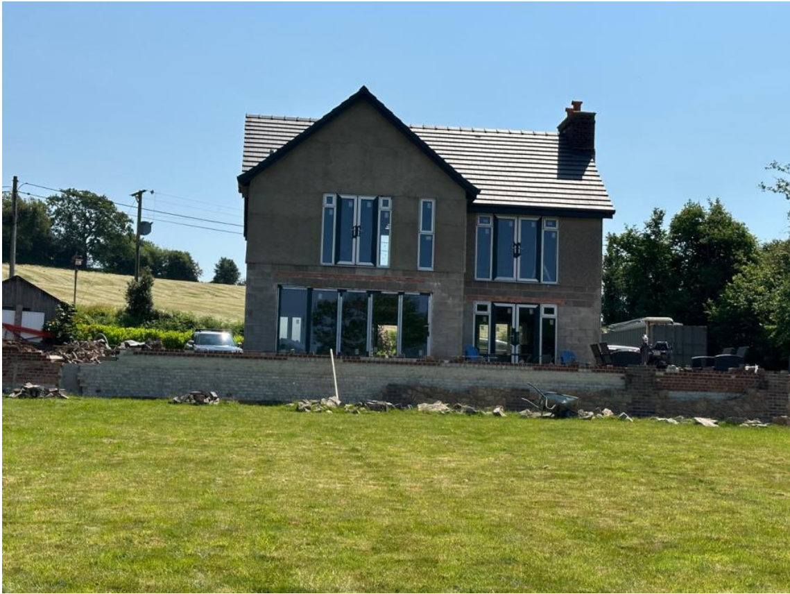
Rear elevation (north west)
