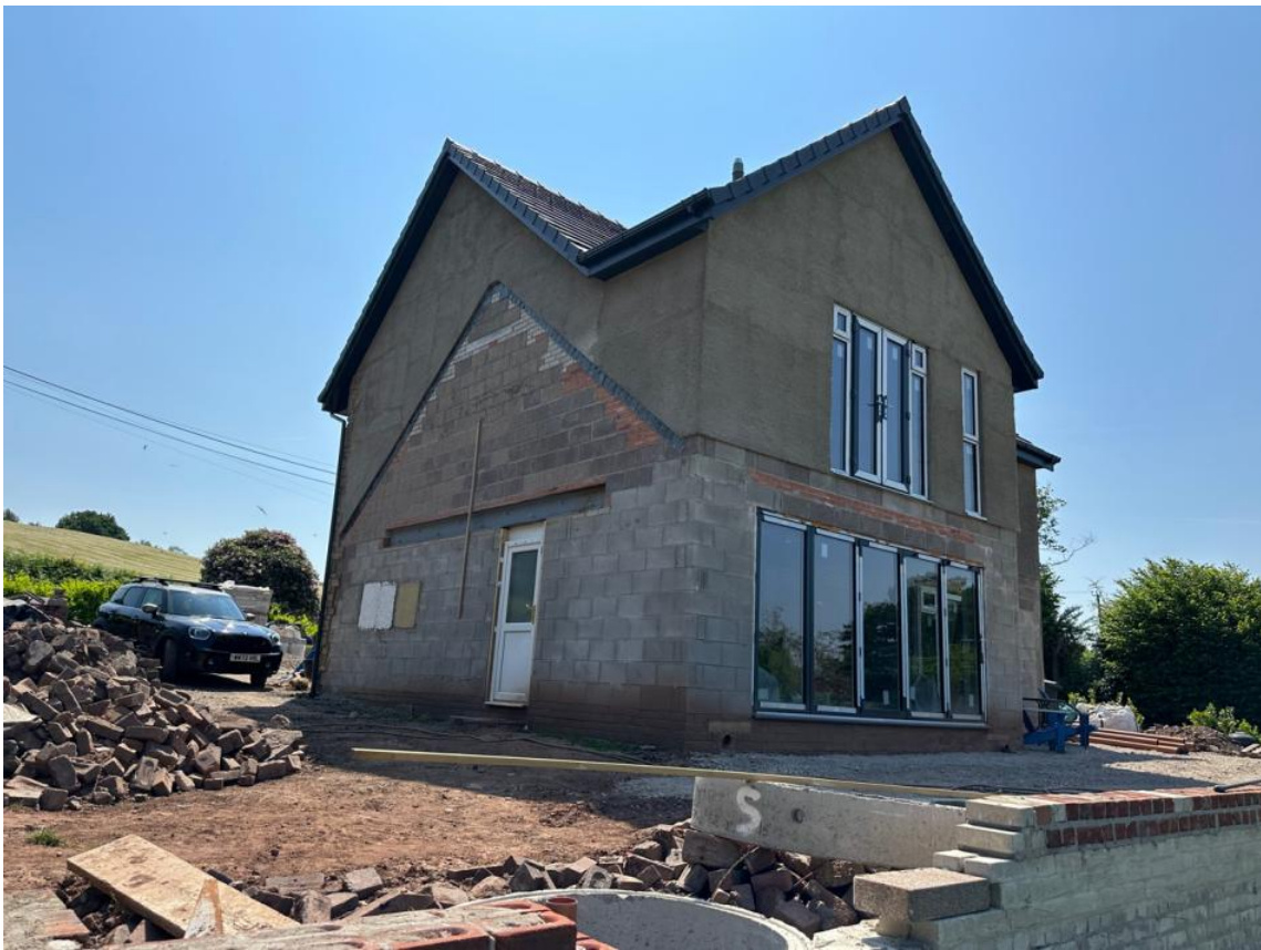
Oblique rear and side elevations(north west)
