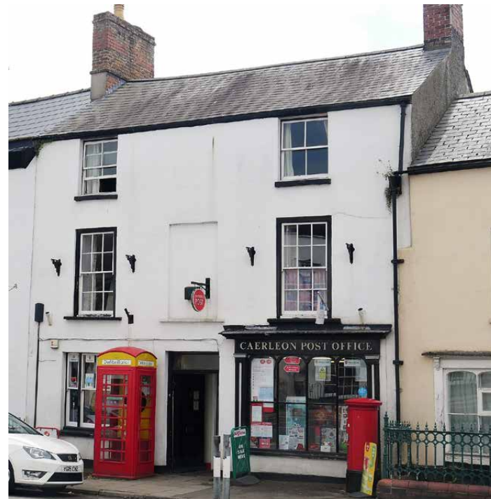
G - Post Office, High Street, July 2021 (source: 'britishlistedbuildings.co.uk')
