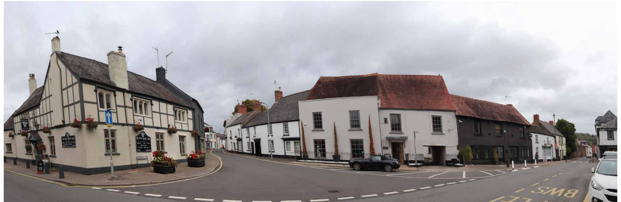
Panoramic view of northern face of High Street, looking down Cross Street, with 9, High Street directly in front in the centre, with the brown render
