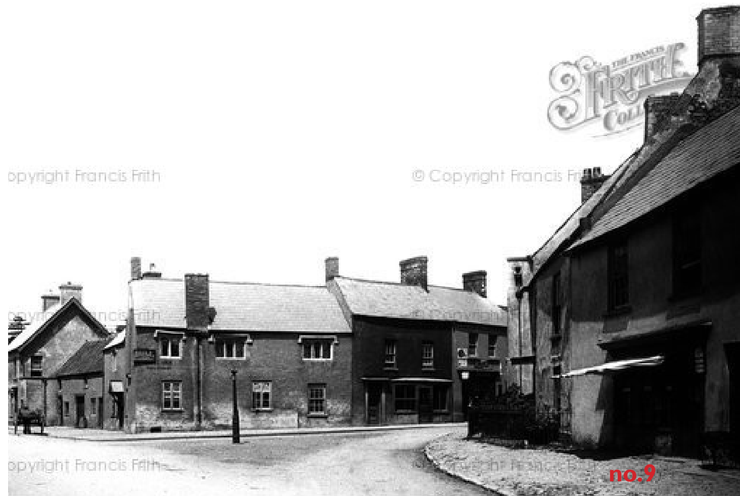
1899 view towards 9 High Street from the south east (source: 'francisfrith.com')
