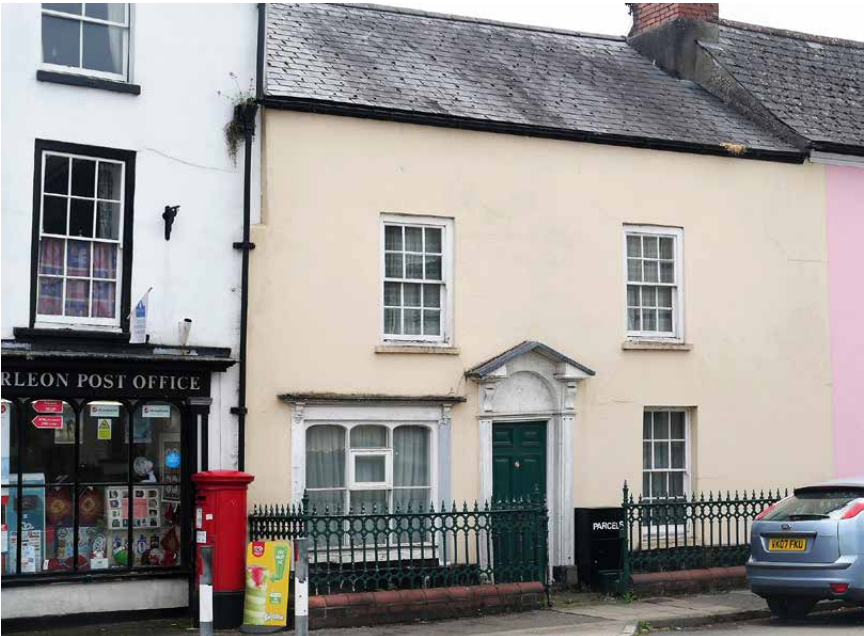
J - No 32 including attached railings, June 2021 (source: 'britishlistedbuildings.co.uk')
