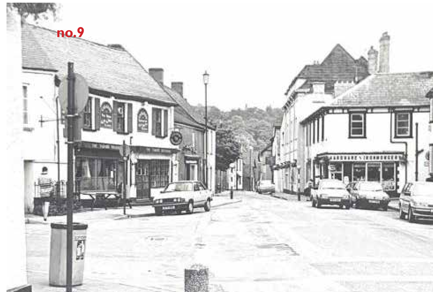
1992 view towards 9 High Street (source: 'southwalesargus')
