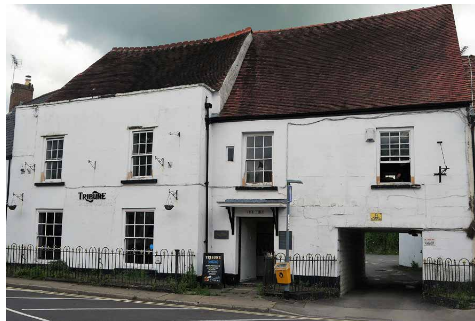
A - The Firs with attached railings, June 2021 (source: 'britishlistedbuildings.co.uk')
