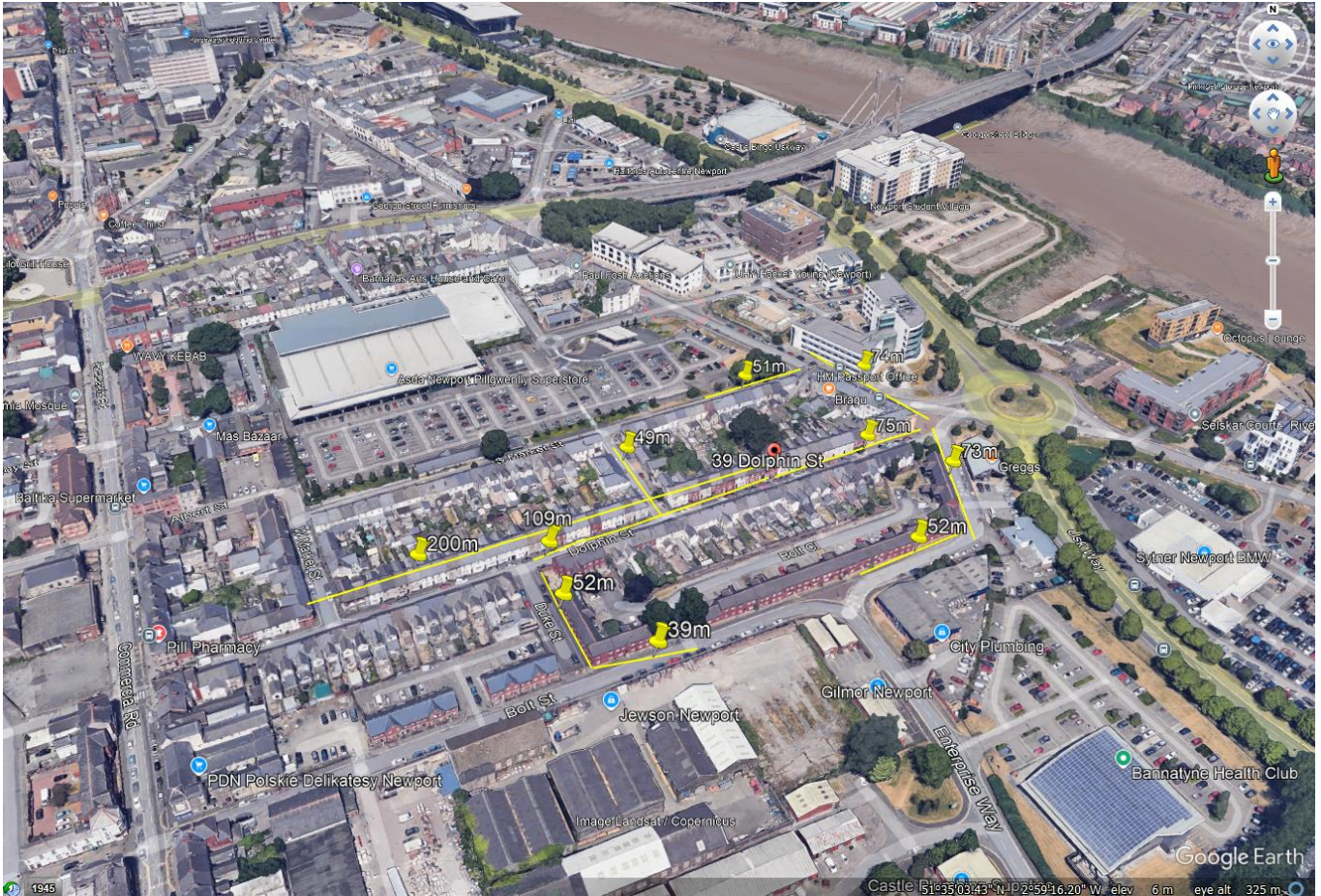
AERIAL PHOTO SHOWING AREA OF SURVEY, WITH DIMENSIONS
