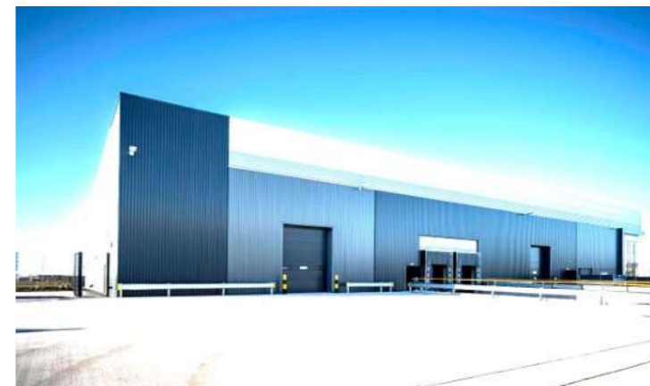
Photograph from within the service yard
