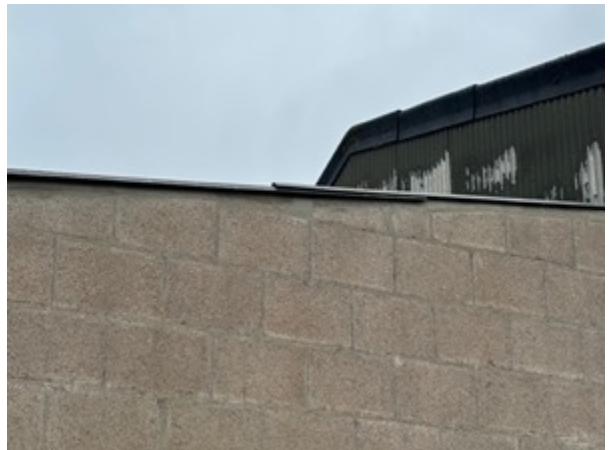
Photo 10: Gaps Under The Roof of Lean-to Extension
