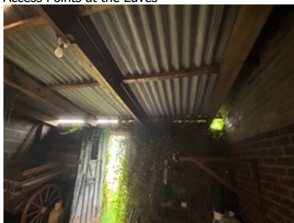
Photo 12: Interior of Lean-to Extension, Showing Access Points at the Eaves
