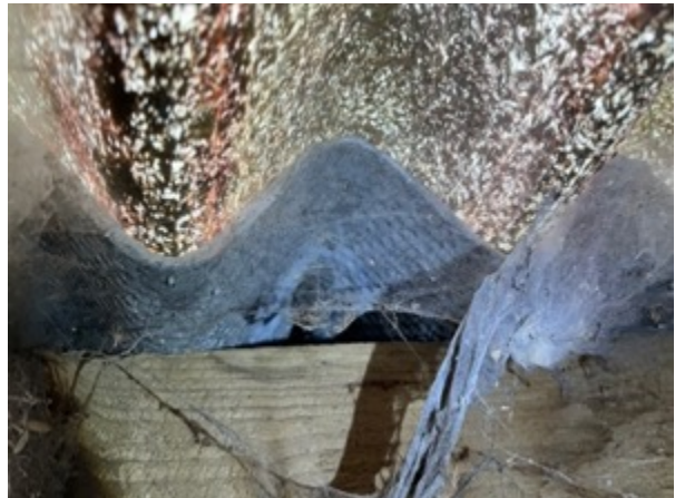
Photo 4: Gaps Underneath The Plastic Sheeting
