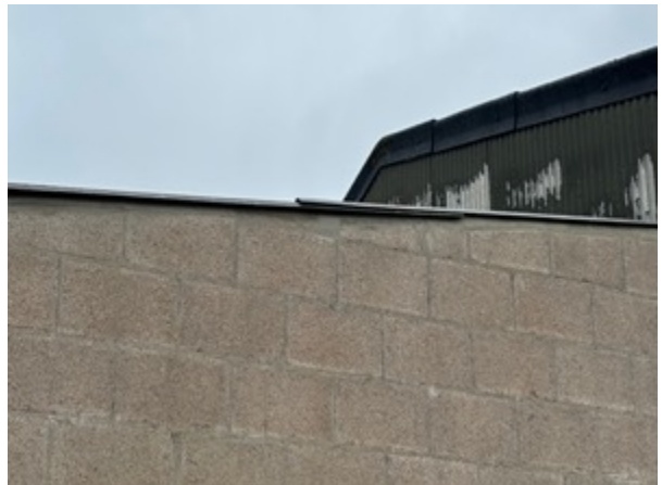
Photo 10: Gaps under the Roof of Lean-to Extension
