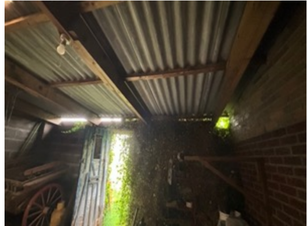
Photo 12: Interior of Lean-to Extension, showing Access Points at the Eaves
