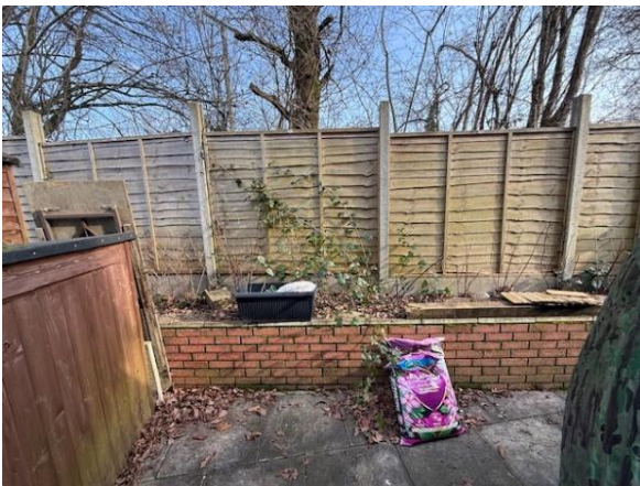
Above image shows the existing low garden retaining wall.
