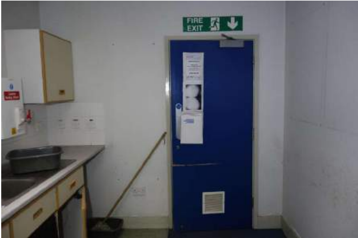
Plate 50: View looking E in GF Room 19.
