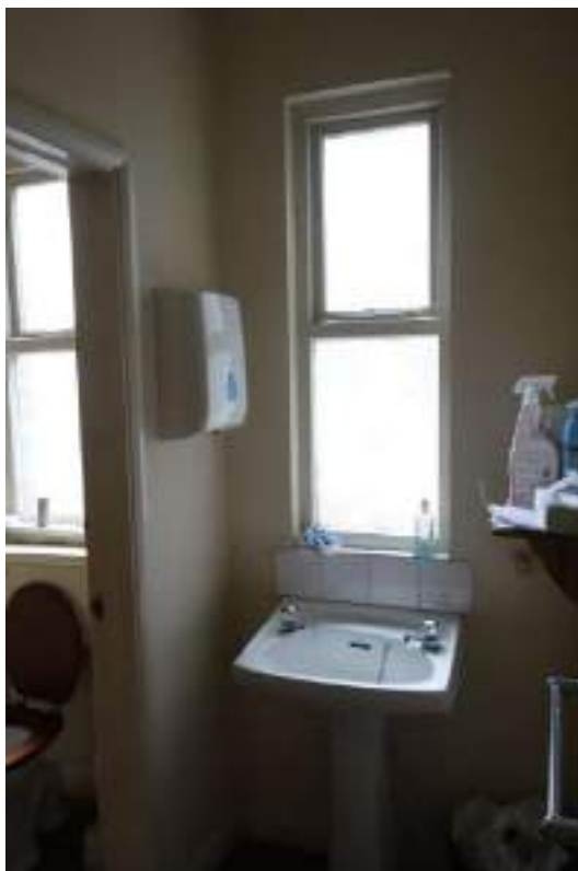
Plate 129: View looking SSE in FF Room 16a, towards two casement windows.
