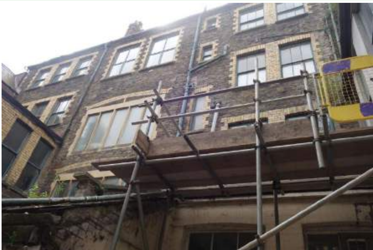
Plate 24: View looking up towards the N-facing elevation of the courtyard.
