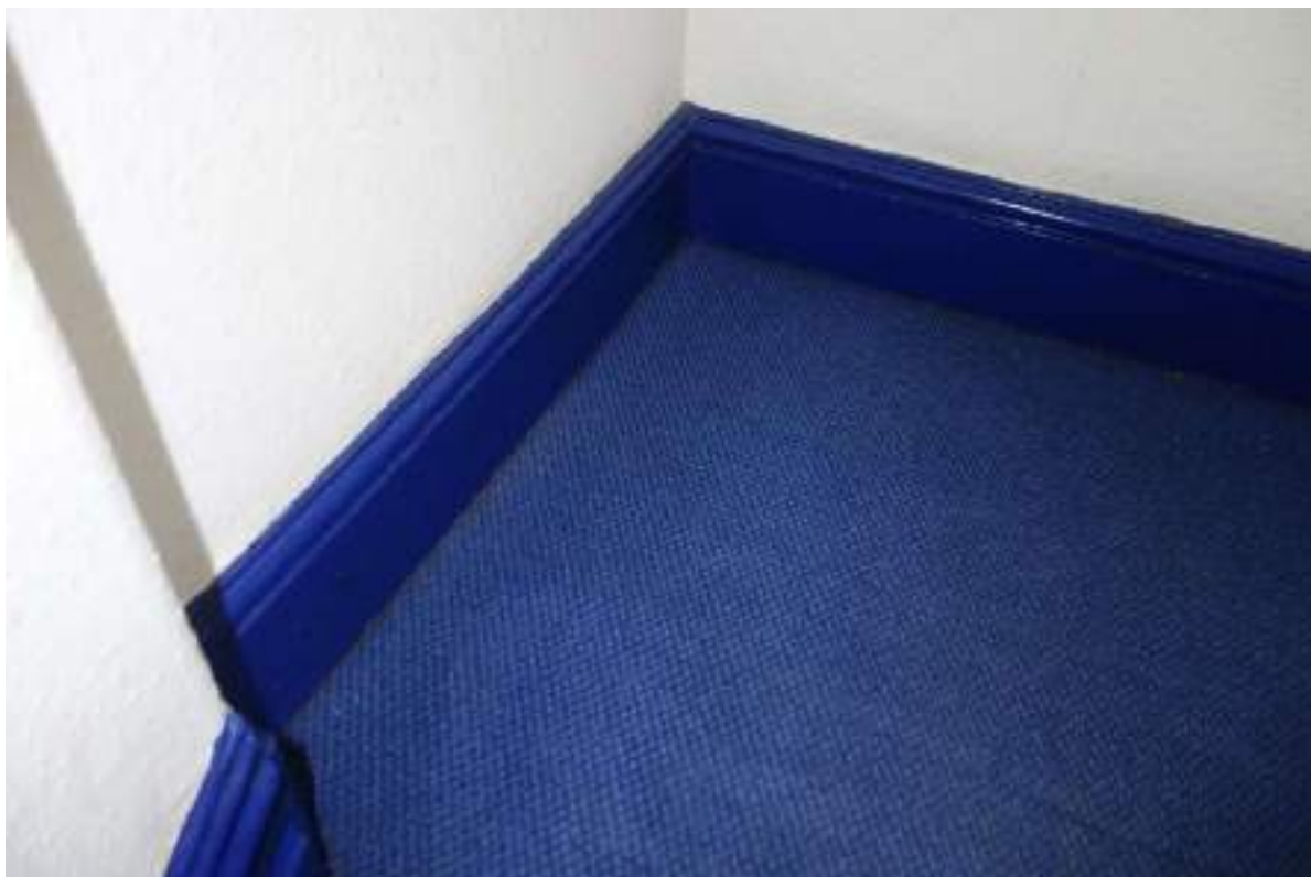
Plate 206: View looking SW at the top of the stairs to TF Room 14, towards the skirting boards.
