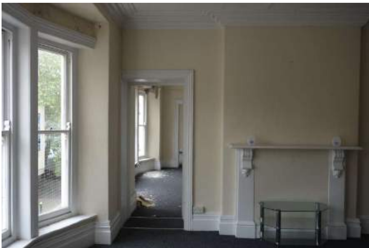
Plate 155: View looking W in SF Room 6, towards a mantel piece and a deep doorway with architrave.
