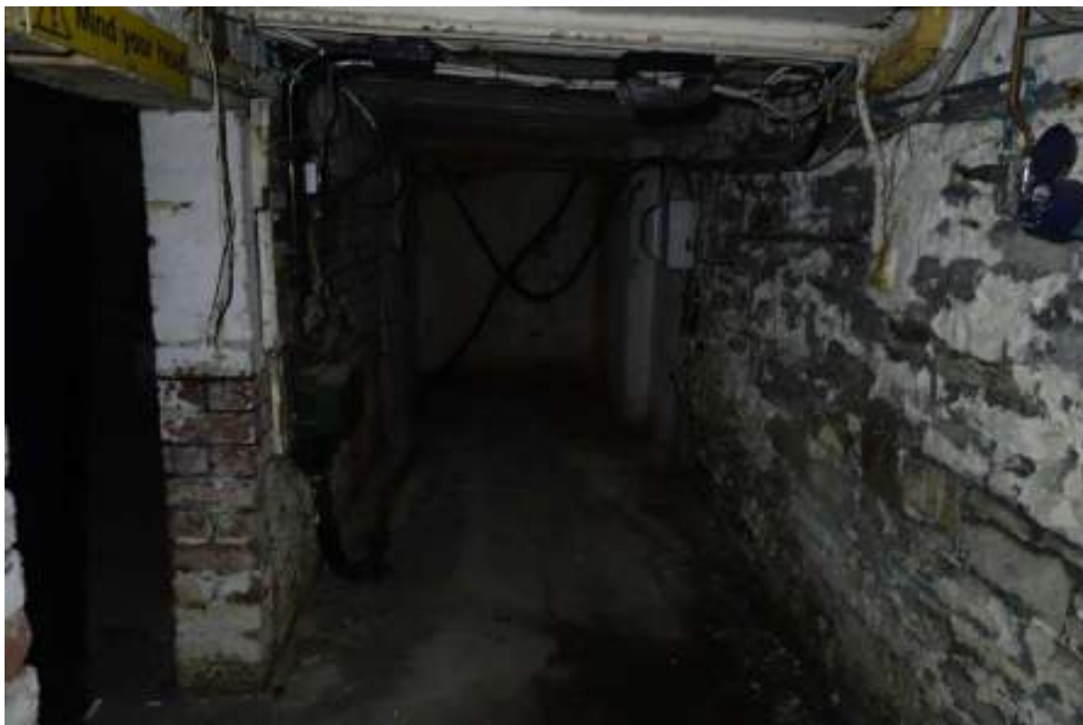
Plate 55: View looking S in the basement's first (W-most) compartment.
