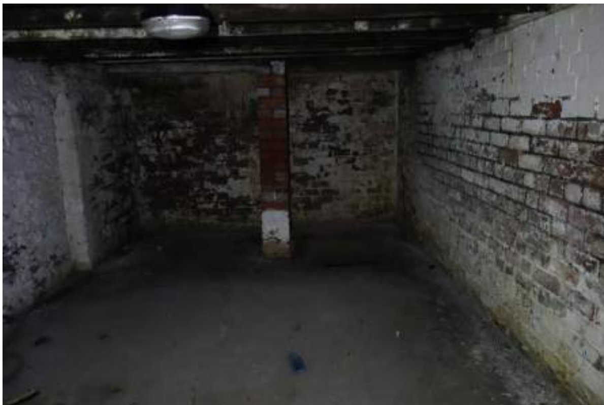
Plate 56: View looking S in the basement's second compartment.
