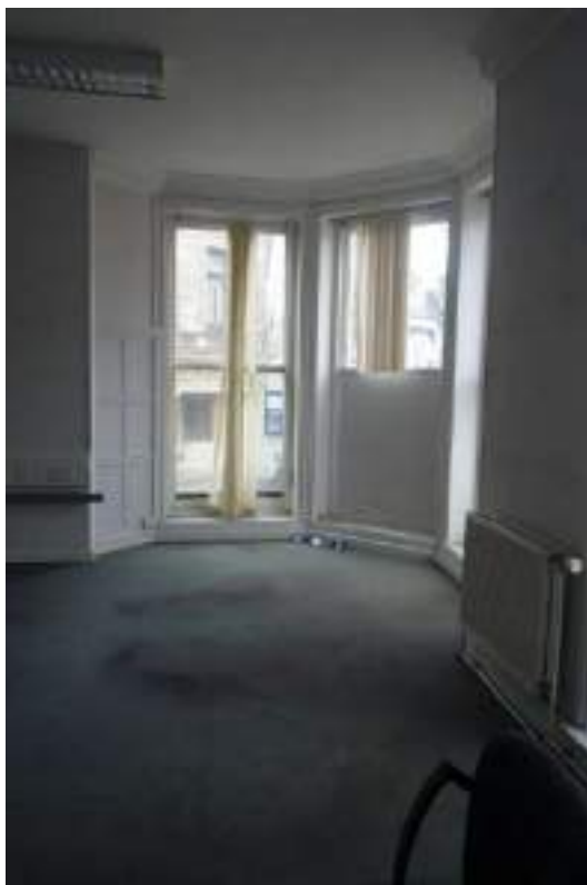
Plate 101: View looking E in FF Room 8, towards the windows of the corner bay and an area of wooden panelling.
