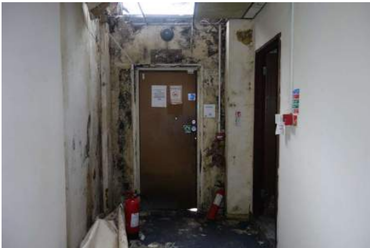
Plate 18: View looking WSW along GF Room 5.
