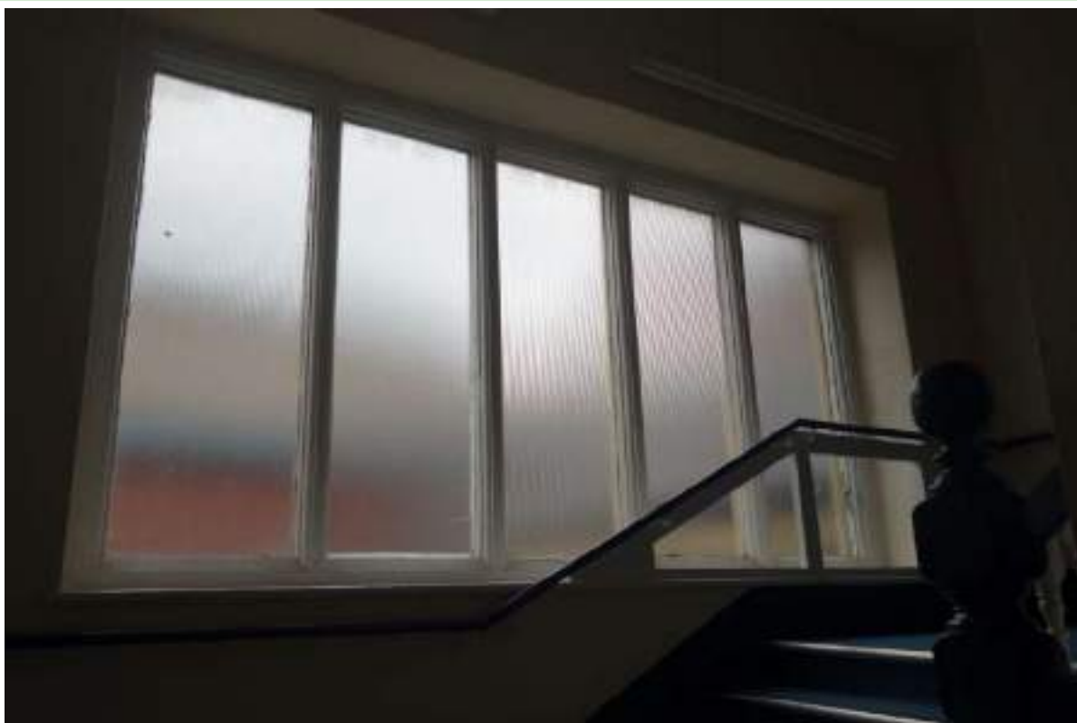
Plate 131: View looking NNE across the centre flight of the main staircase (FF to SF), towards the windows.
