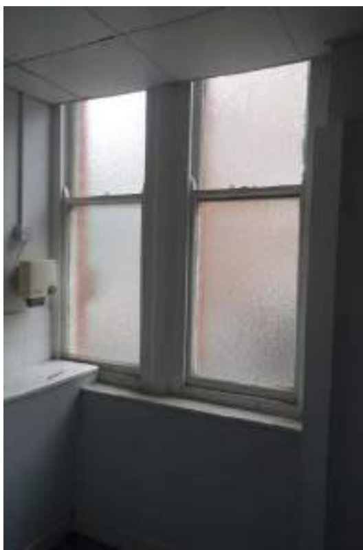
Plate 98: View looking E, towards two sash windows in FF Room 7.
