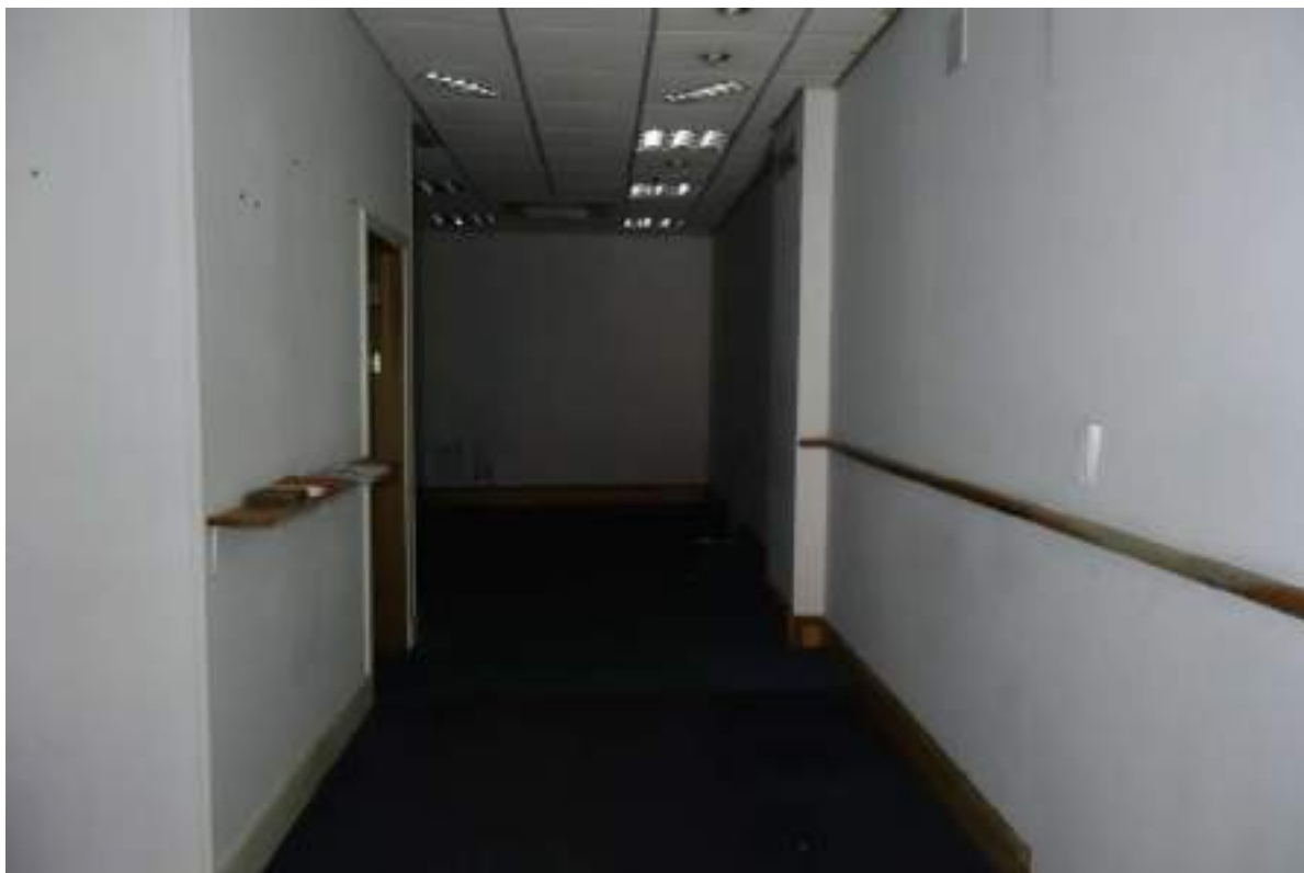
Plate 46: View looking N across GF Room 16.
