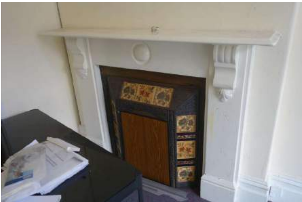
Plate 117: View looking NE in FF Room 12c, towards a wrought-iron fireplace with tiled panels.
