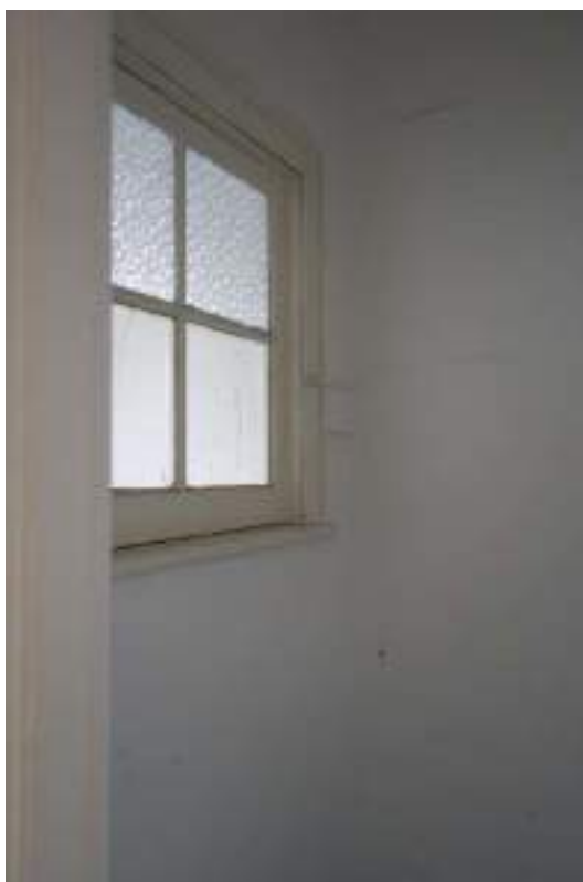
Plate 203: View looking ENE in TF Room 12a.
