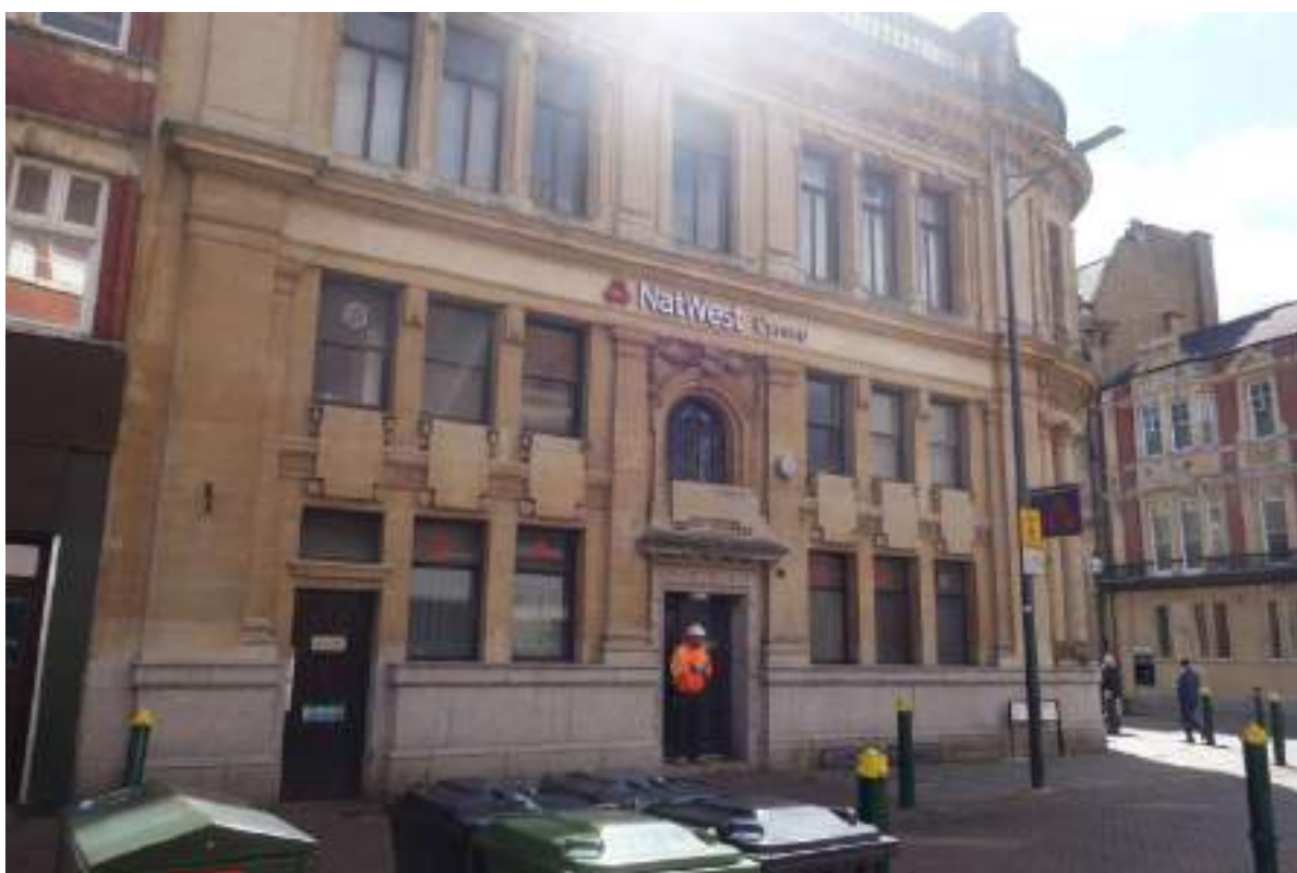
Plate 209: View looking SE towards the National Westminster Bank, along Cambrian Road.
