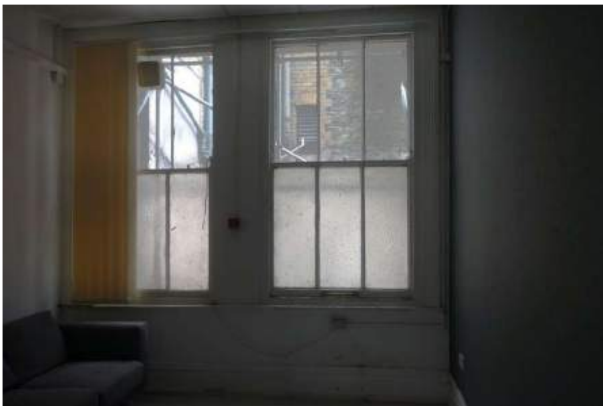
Plate 43: View looking N in GF Room 14, towards two sash windows.
