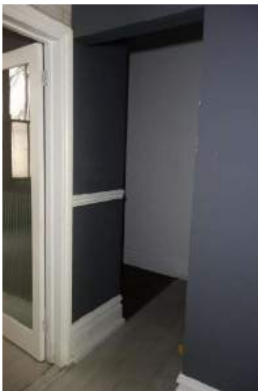
Plate 41: View looking NE in GF Room 13, towards a section of dado rail, moulded skirting board, and architrave.
