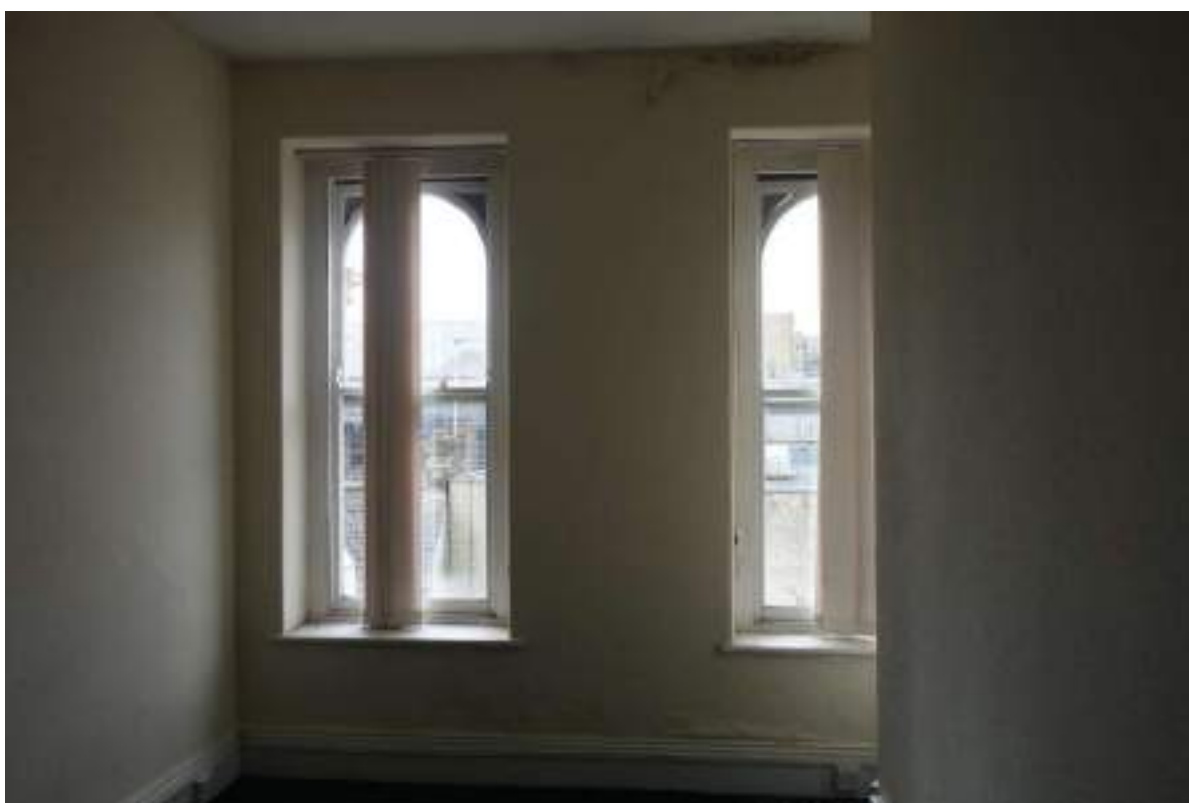
Plate 183: View looking N in TF Room 3, towards two faux-arched sash windows.
