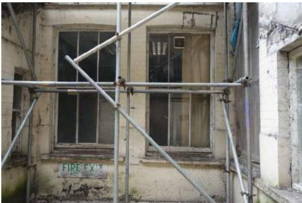
Plate 23: View looking S towards the N-facing courtyard elevation.
