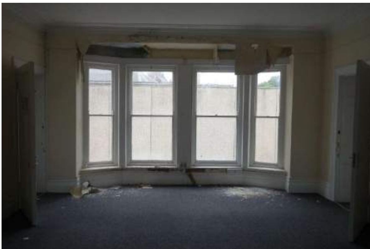
Plate 157: View looking S in SF Room 7.
