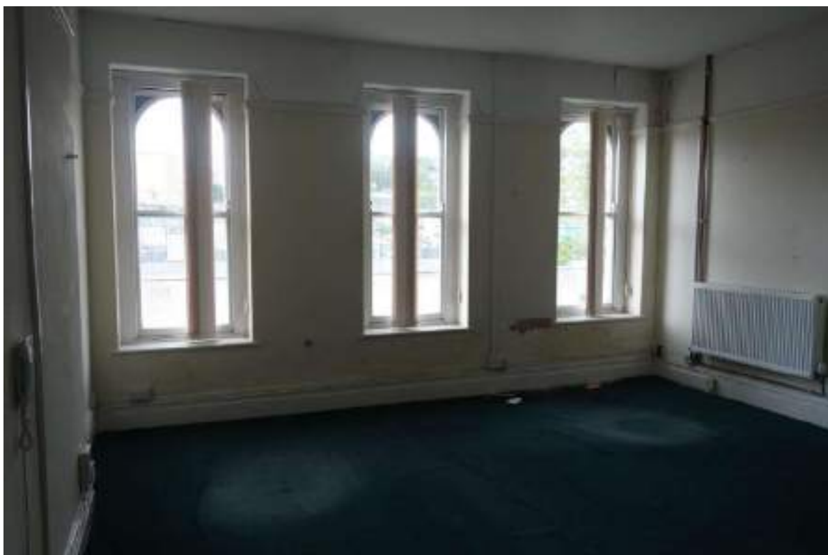
Plate 196: View looking N into TF Room 10, towards three faux-arched sash windows.
