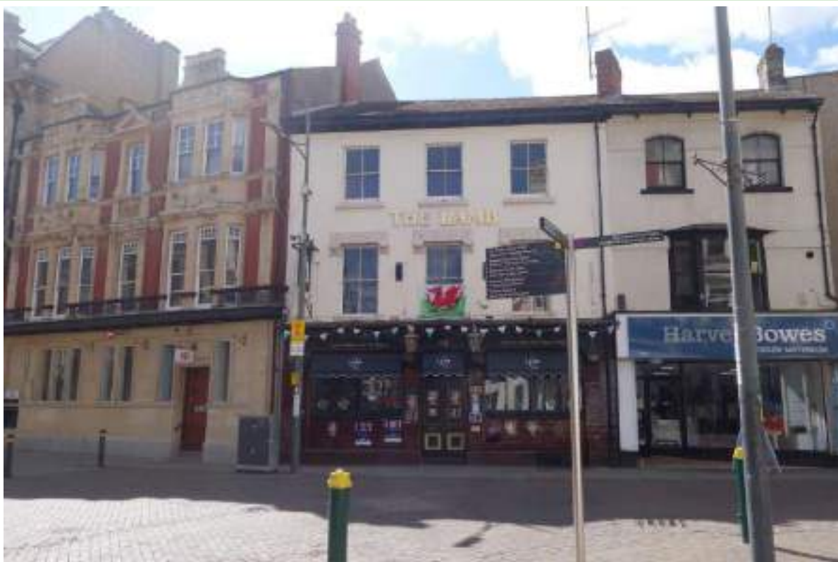
Plate 208: View looking NNE towards The Lamb Public House.
