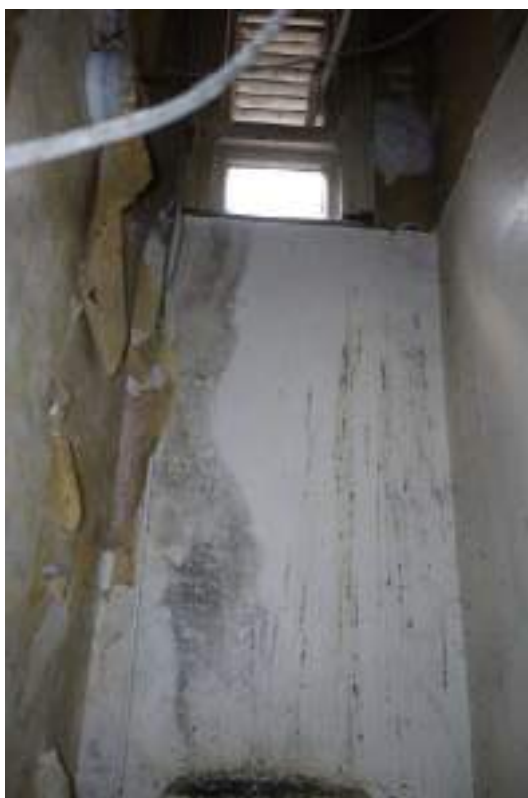
Plate 32: View looking SSE in GF Room 10, towards a louvre window.
