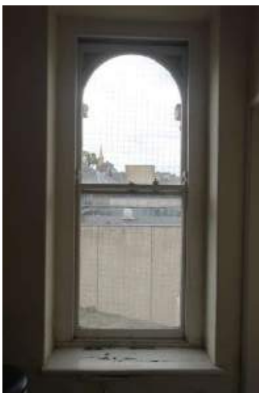
Plate 194: View looking S in TF Room 9, towards a faux-arched sash window.
