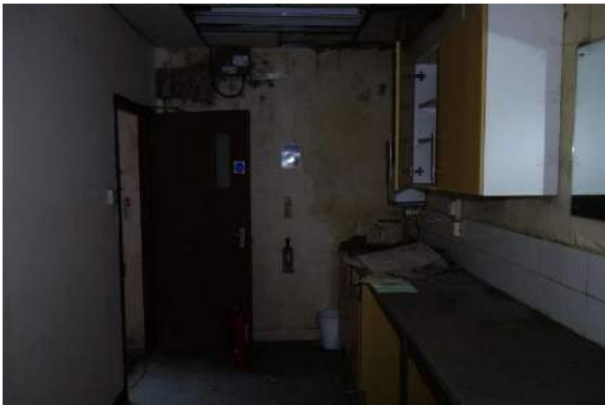
Plate 20: View looking WSW across GF Room 7.
