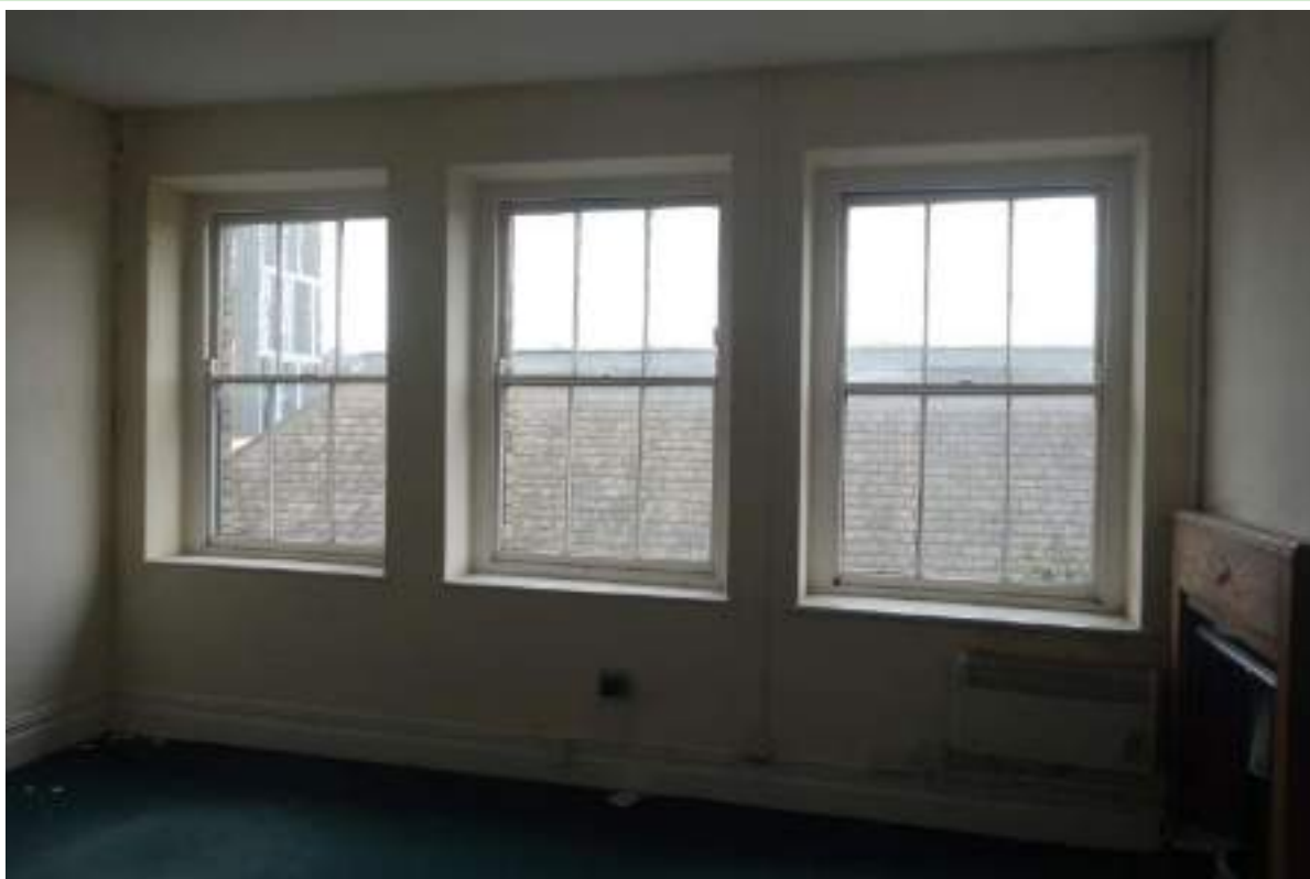
Plate 199: View looking NNW in TF Room 12, towards three sash windows.
