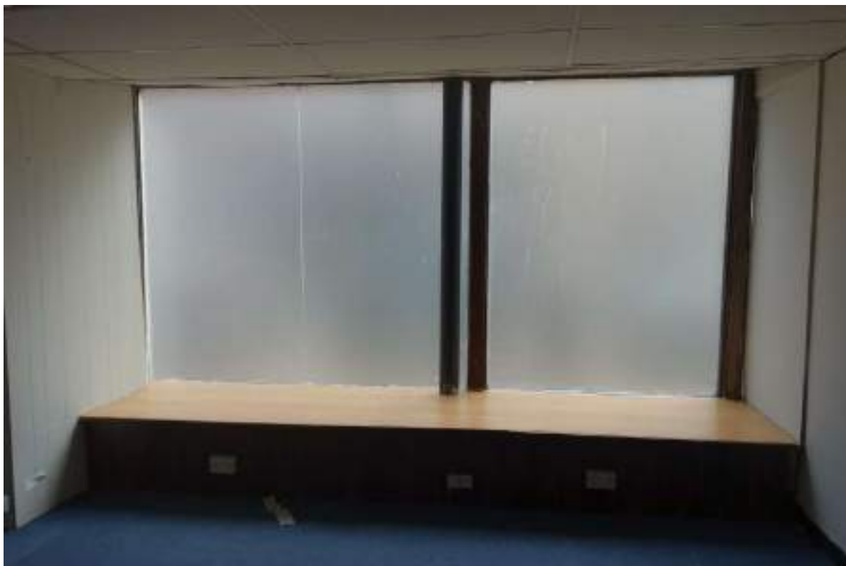
Plate 16: View looking E in GF Room 4.
