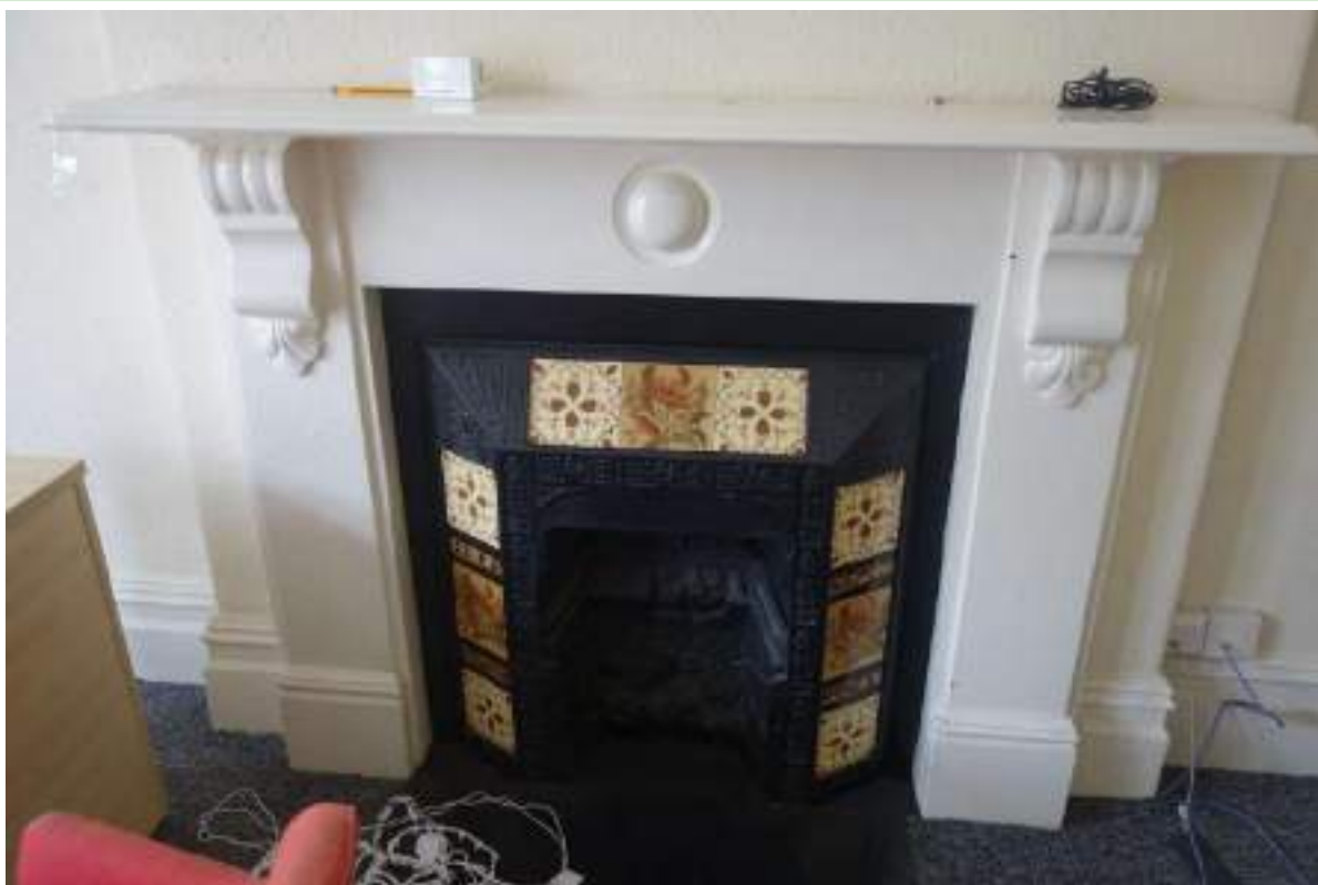
Plate 112: View looking W in FF Room 11, towards a wrought-iron fire place with tiled panels.
