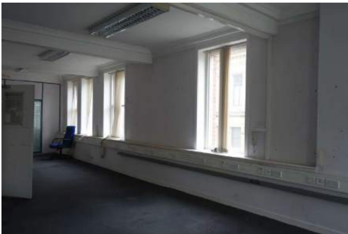
Plate 102: View looking NE along FF Room 8.
