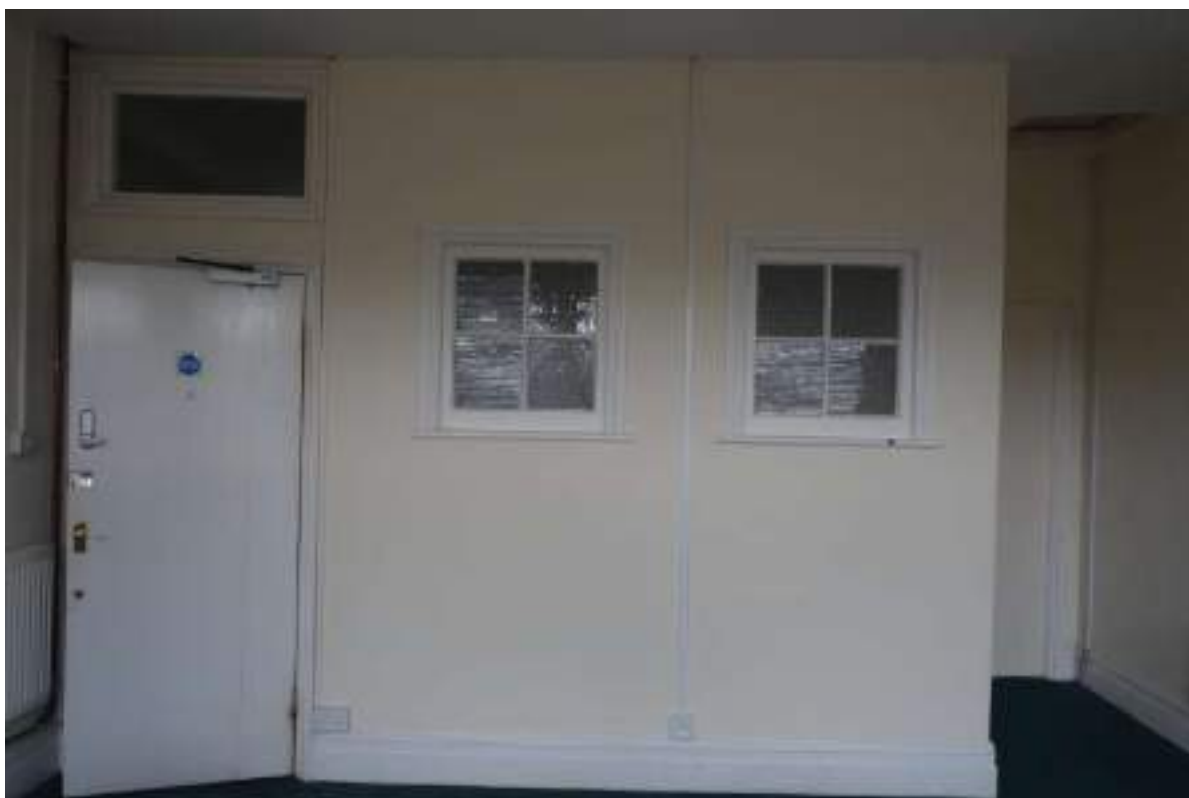
Plate 200: View looking S in TF Room 12, towards two interior windows.
