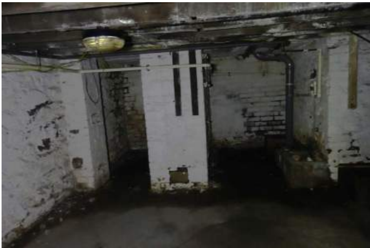
Plate 57: View looking N in the basement's second compartment.
