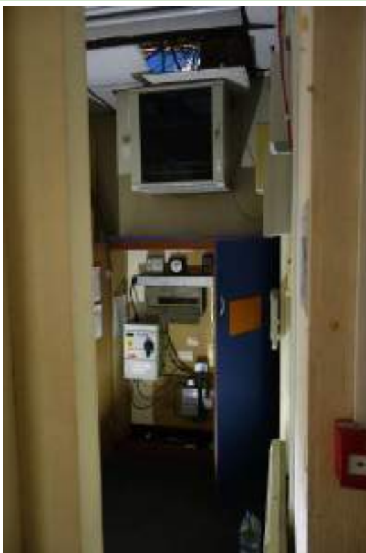
Plate 12: View looking NE in GF Room 2.
