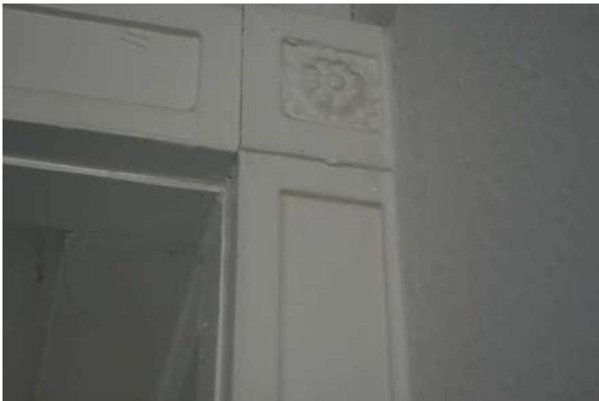
Plate 95: View looking W in FF Room 6, showing a close-up of the architrave's corner block.
