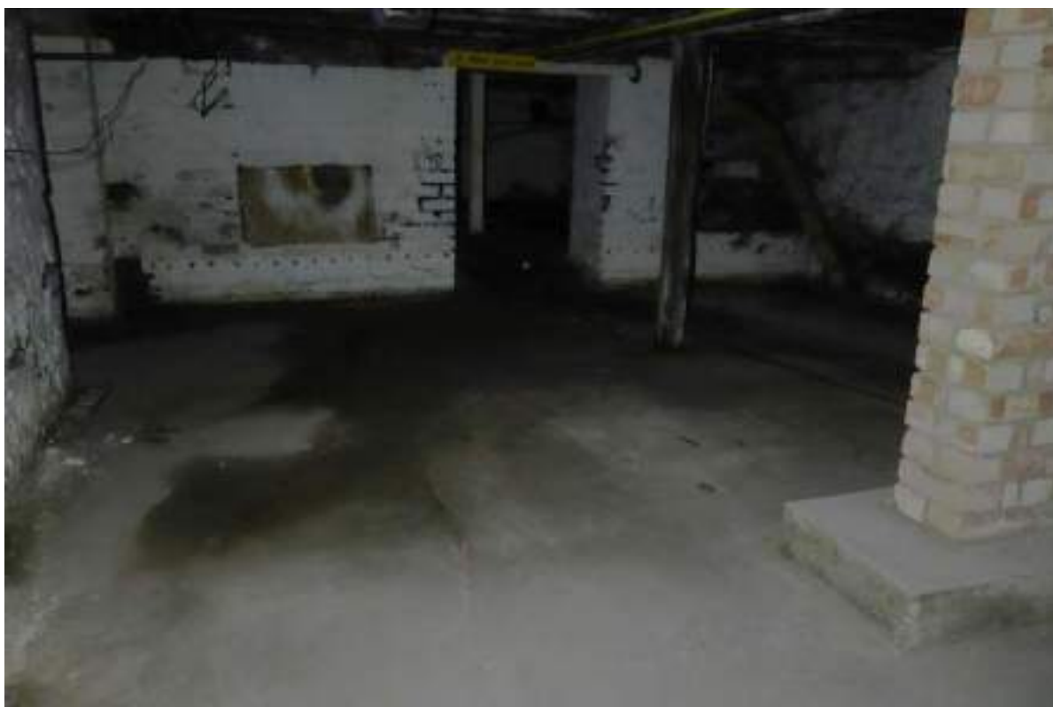
Plate 58: View looking NE in the basement's third compartment.
