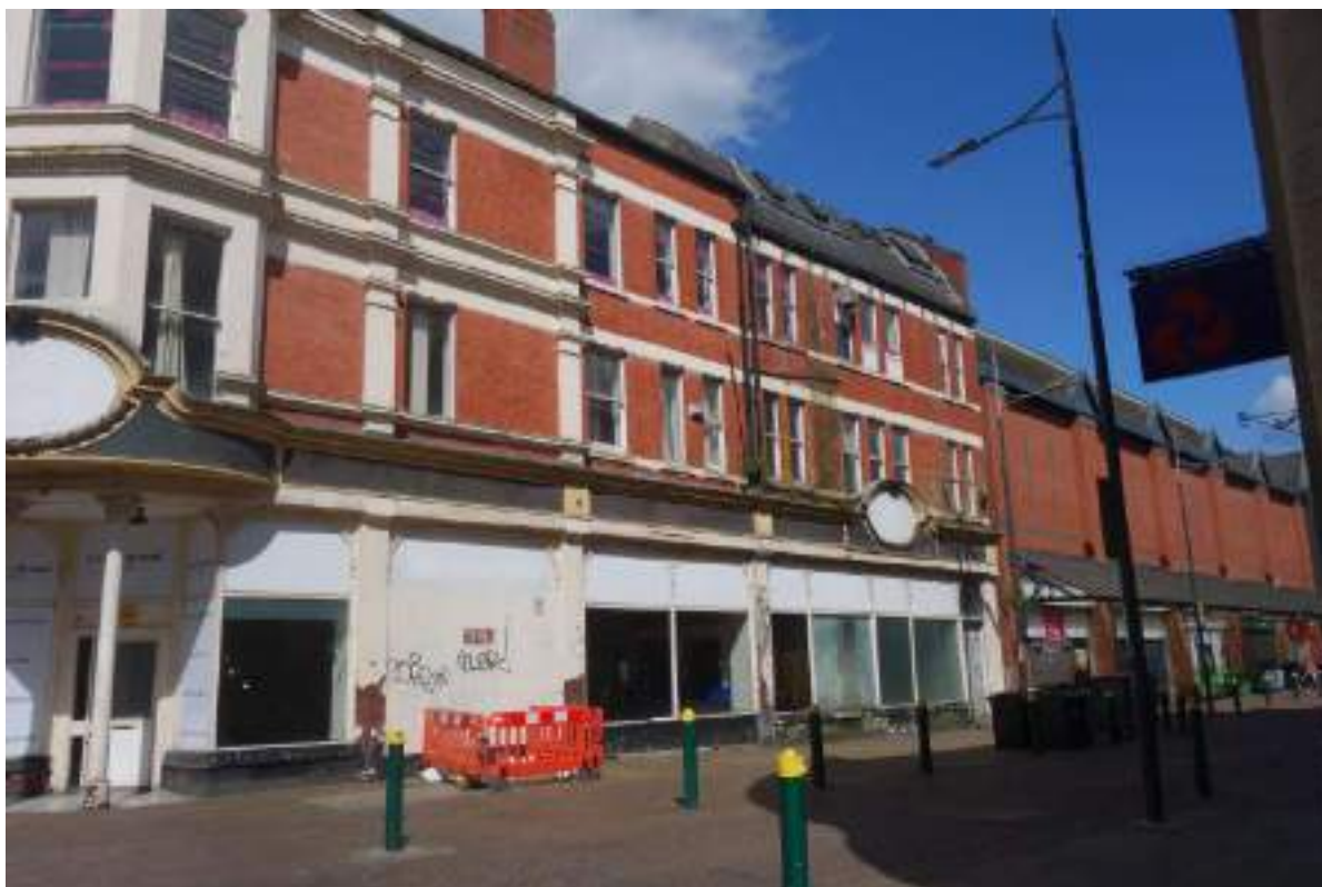
Plate 6: View looking WNW towards Tredegar Chambers' Cambrian Road elevation.
