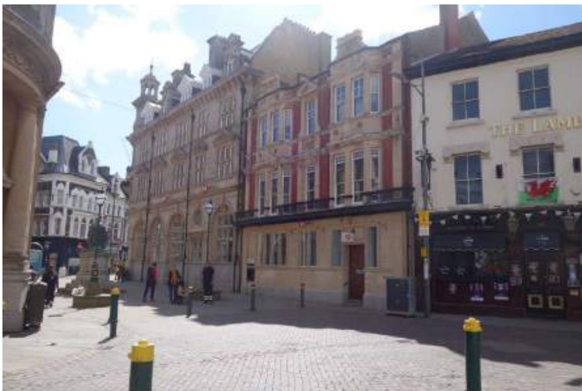
Plate 211: View looking NE towards the Bridge Street elevation of HSBC (formerly Midland Bank).
