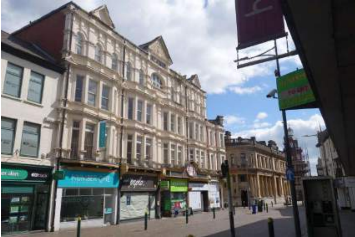
Plate 1: View looking ENE towards Tredegar Chambers' Bridge Street elevation.
