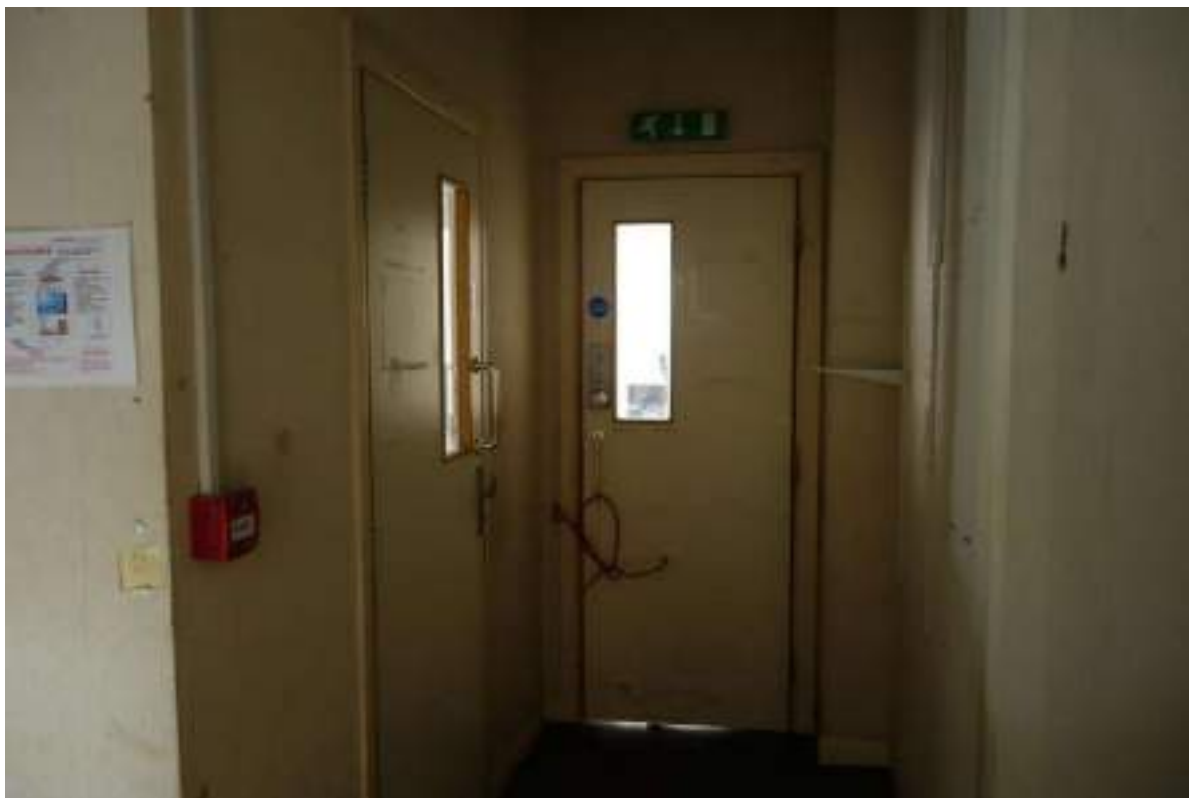
Plate 11: View looking S along GF Room 2.
