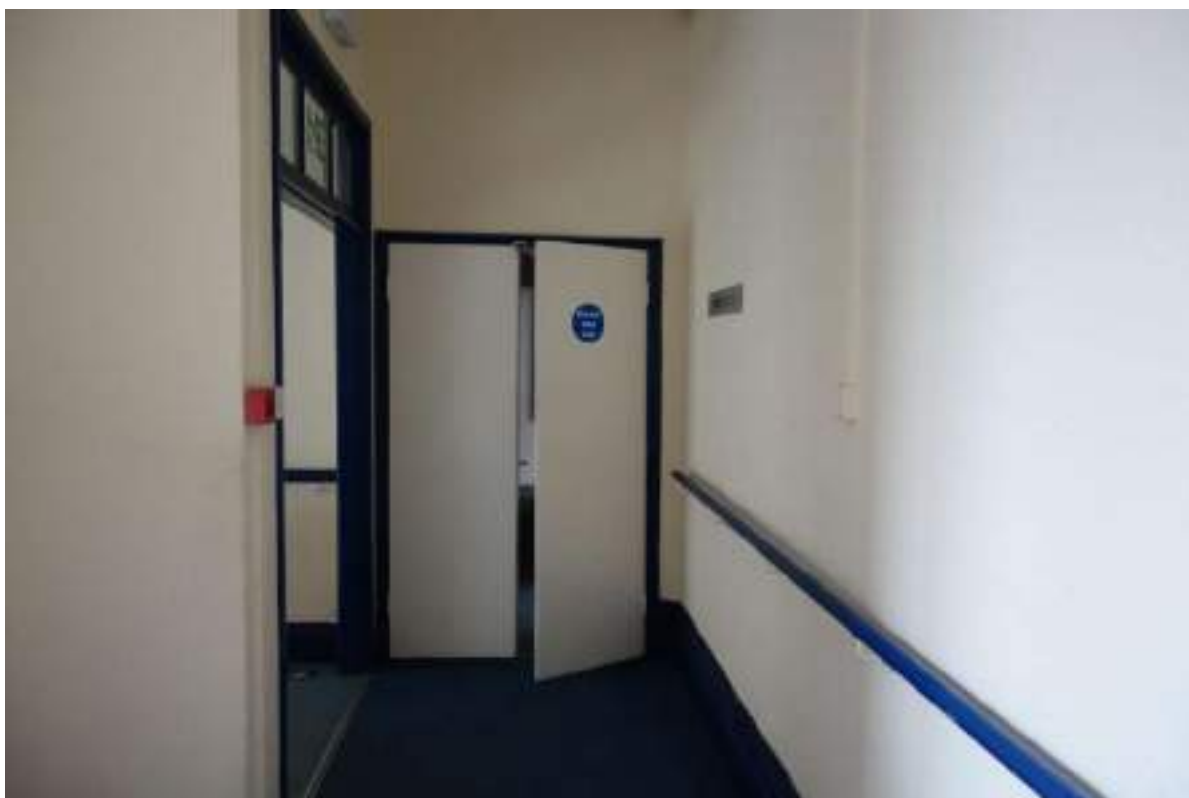
Plate 77: View looking E along FF Room 1.
