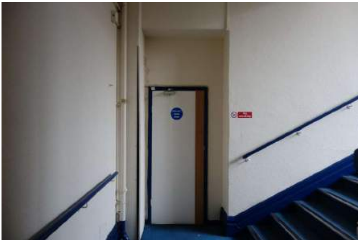
Plate 78: View looking W along FF Room 1.
