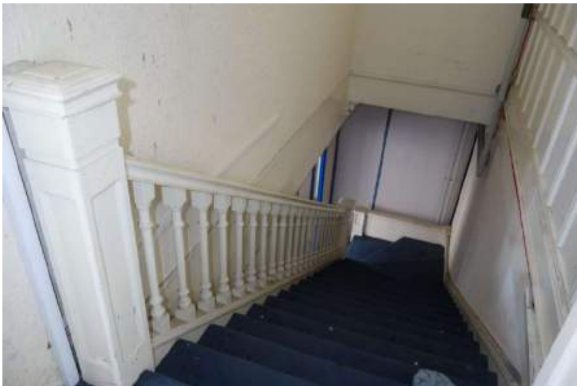
Plate 103: View looking S, down the FF to SF E-bay staircase.
