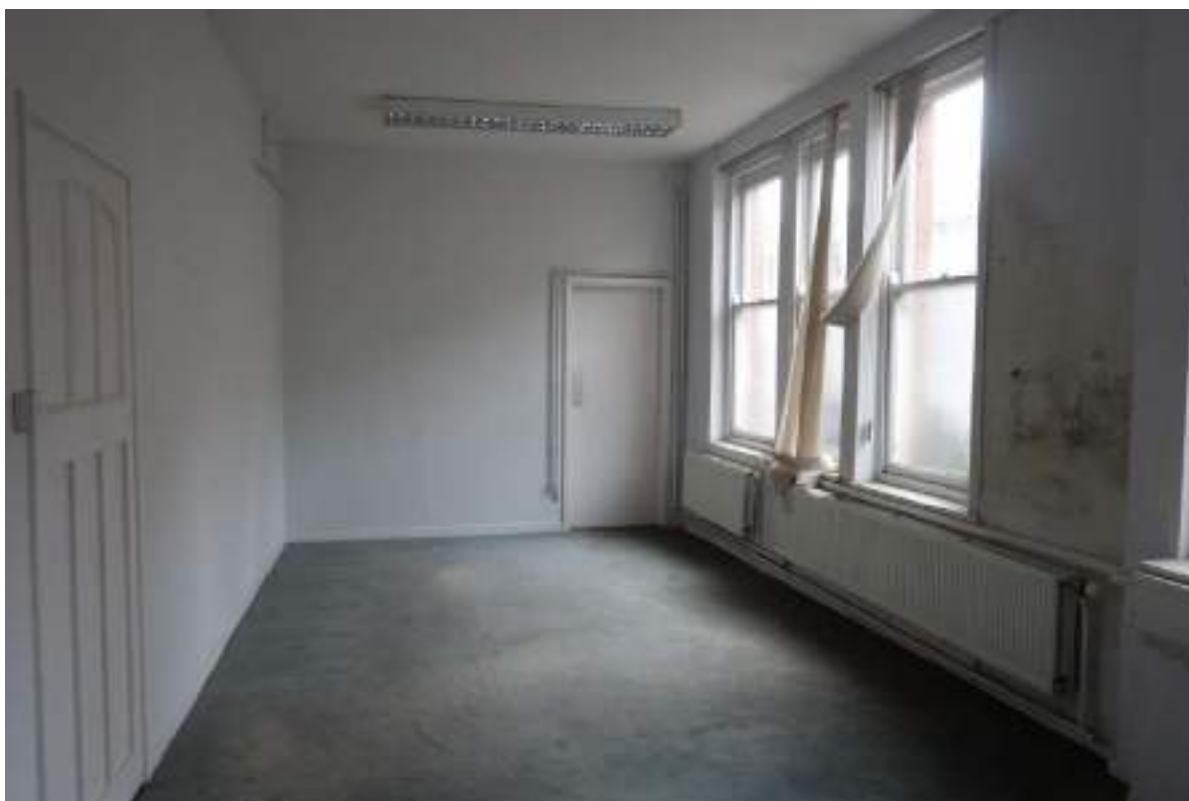
Plate 92: View looking NE in FF Room 6.
