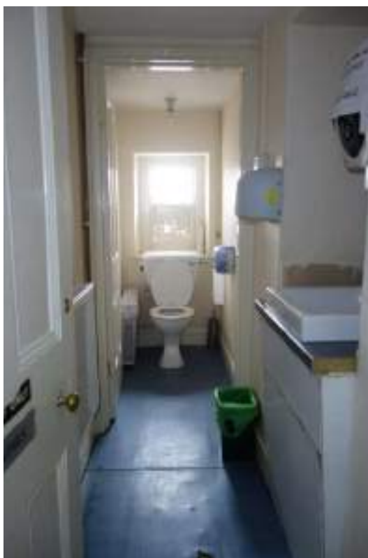
Plate 207: View looking N in TF Room 14, towards a sash window.
