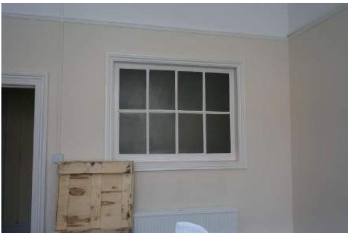
Plate 120: View looking S in FF Room 13, towards an interior window.
