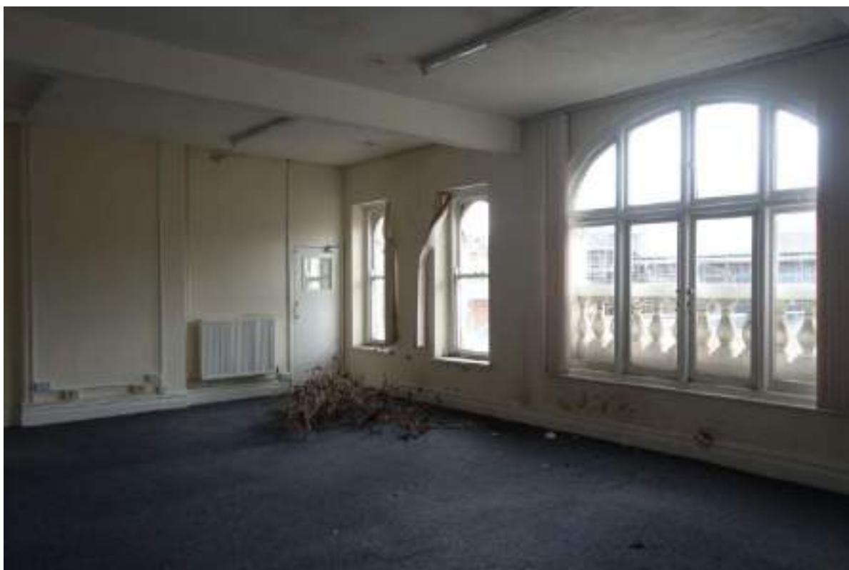
Plate 190: View looking SE across TF Room 8.
