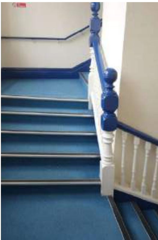
Plate 176: View looking E along the main staircase's (SF to TF) middle flight, showing two newel posts and the stairs' camber.
