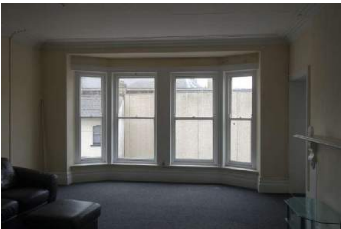
Plate 153: View looking S in SF Room 6.
