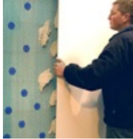
Plaster board being fixed to membrane.
