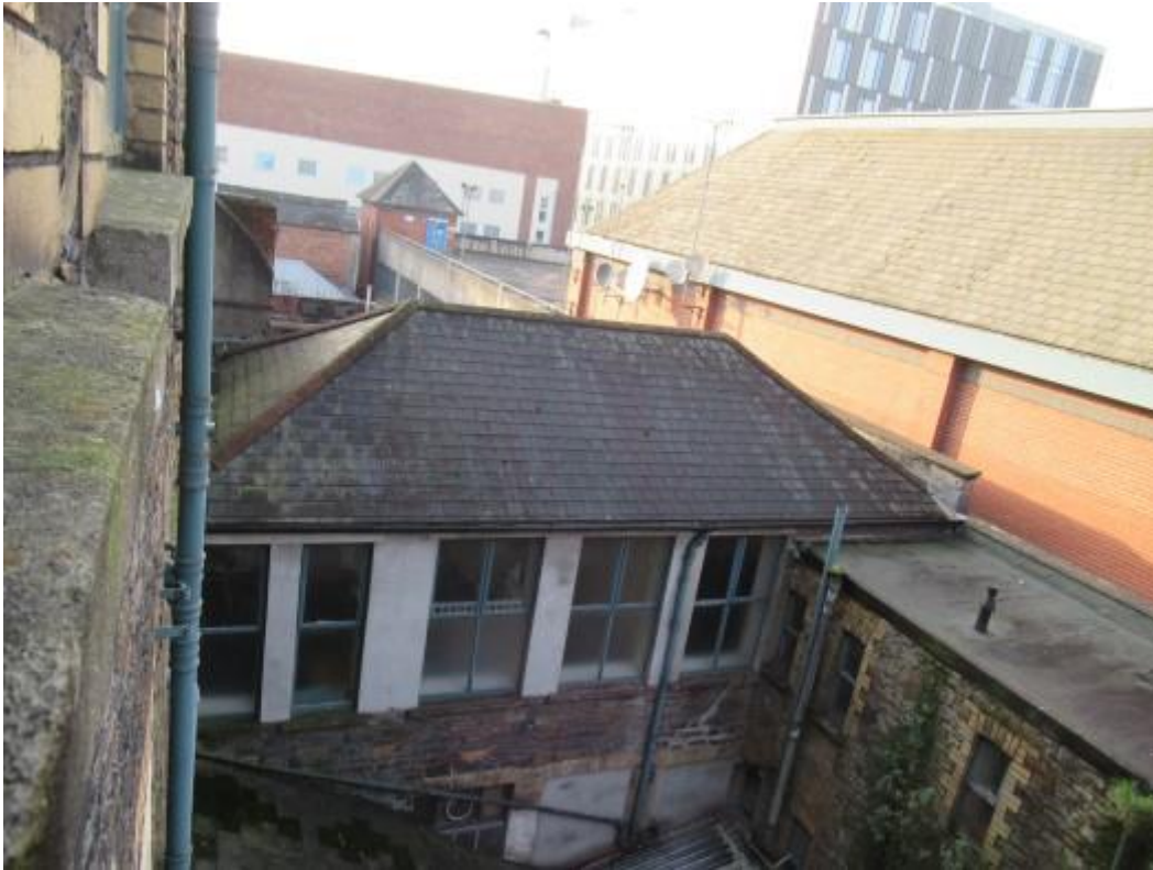
Further illustration of the rear left hand side lower level roof area. The hipped style of the roof is noted.
