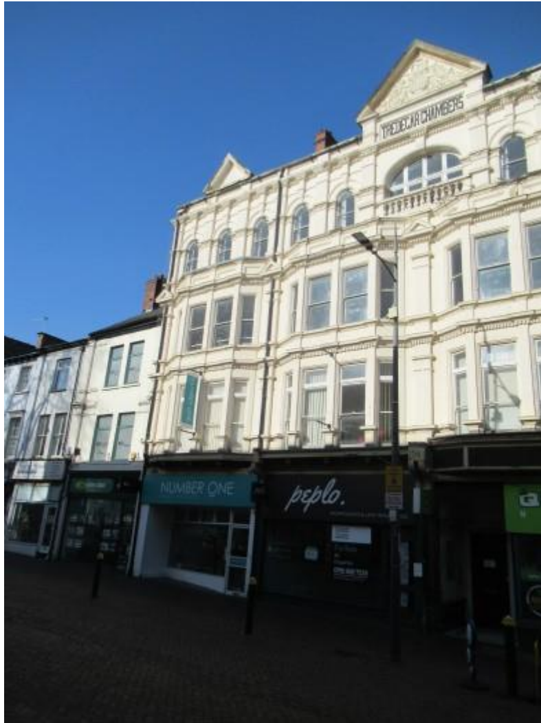
Further illustration of the front elevation. The photograph shows the general condition of the ground floor shop fronts and render and stone walling finishes where extending above.
