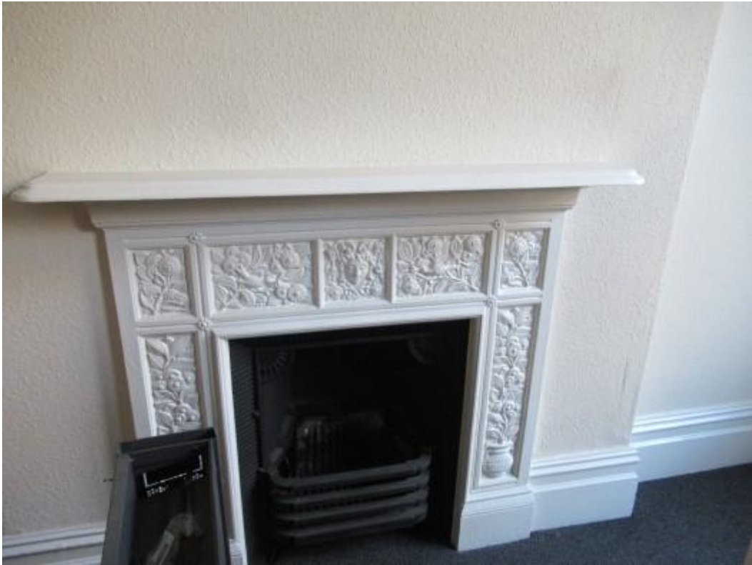
Further illustration of typical cast iron fire grate retained within the property.
