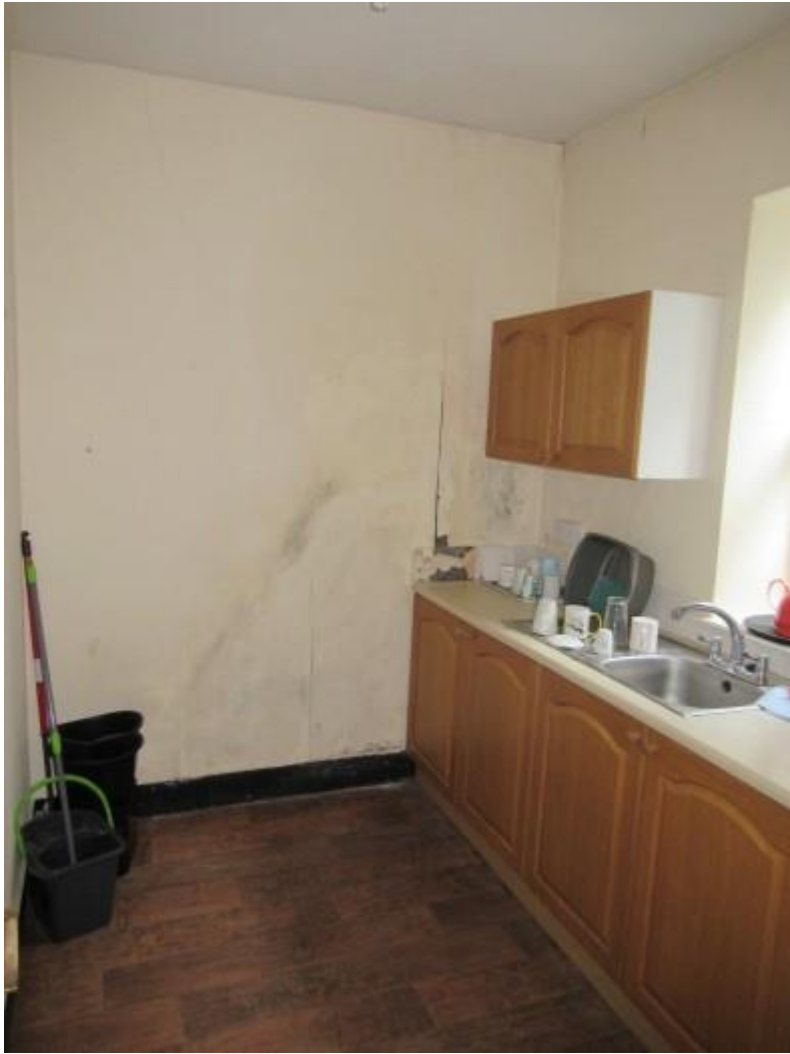
Kitchen accommodation to the first floor to the rear of No. 76.
