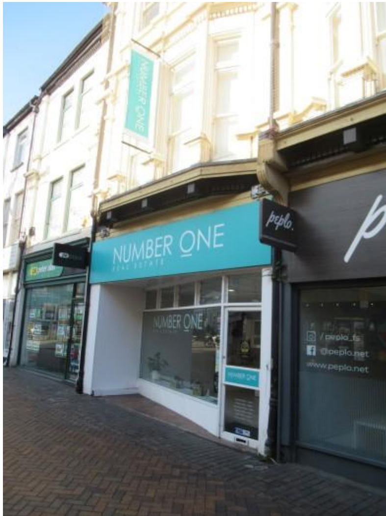
Shop front to ground floor left hand side retail unit. The unit is currently tenanted.
