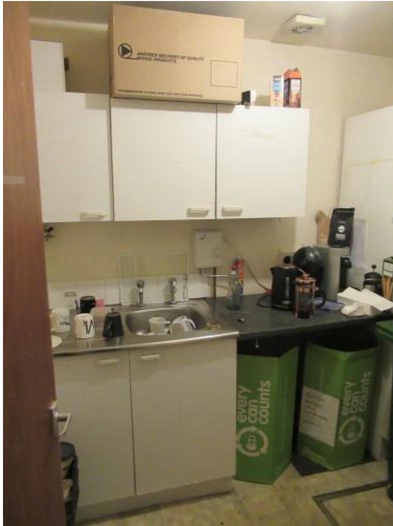
Typical condition of kitchen units to ground floor unit, No. 76.
