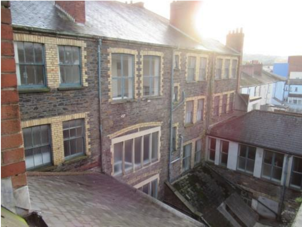
Further illustration of walling to the rear of the main building.
