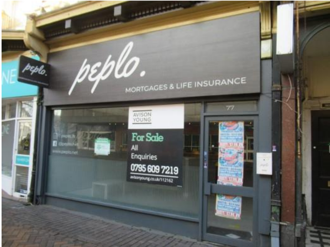
Shop front to No. 77. The photograph also shows the fascia detailing where extending above the shop fronts. There are areas of rot and decay affecting the timbers above. Repair and upgrading work will be required as necessary.
