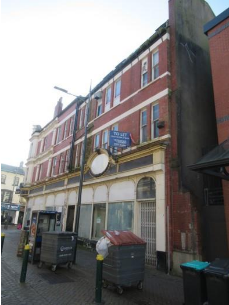
Right hand side elevation as viewed from the rear.
