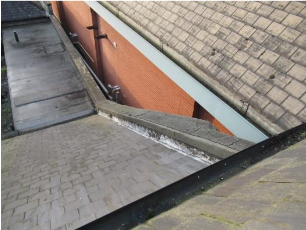
Bitumen felt covering to the parapet coping to the rear.
