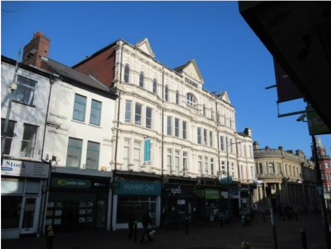
Further illustration of the front elevation. The photograph shows the render and stone detailing to the main elevation. The photograph also shows the bay windows where extending to the first and second floors with small flat roof areas above.
