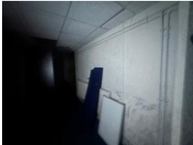
Figure 3 Basement wall for proposed removal (3)
