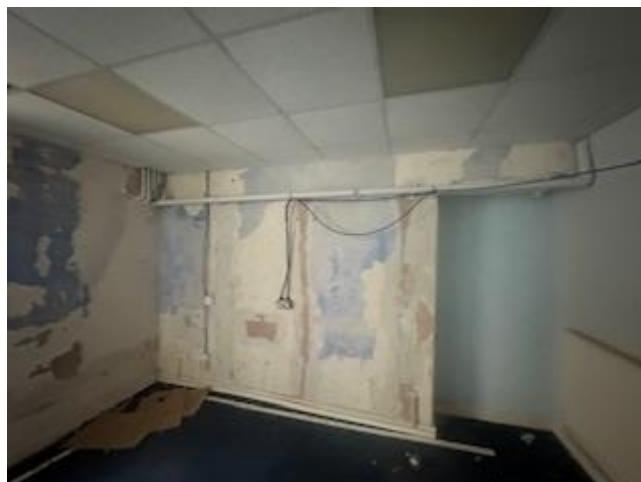
Figure 2 Basement wall for proposed removal (2)
