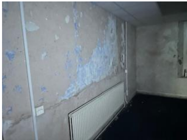
Figure 1 Basement wall for proposed removal (1)
