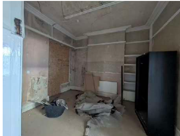
5. Typical room showing extent of surviving fabric and detailing
