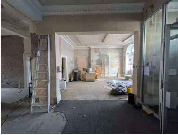
7. Ground entrance lobby and reception
