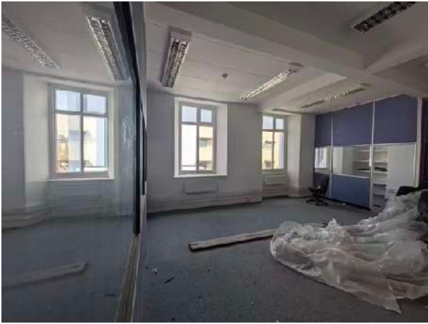
10. First floor office showing typical detailing
