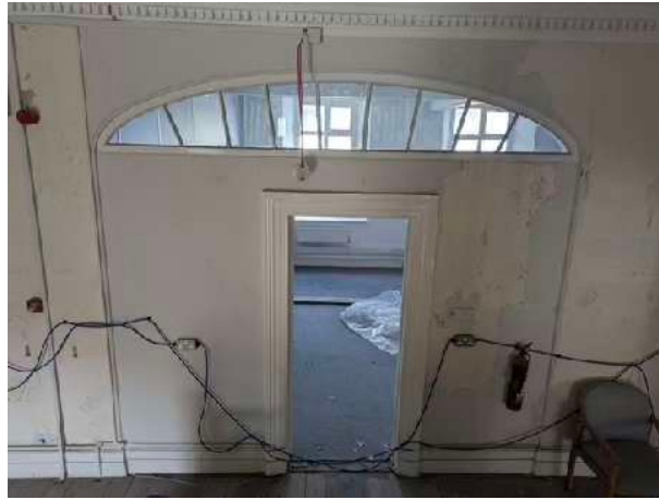
11. First floor landing infill arch
