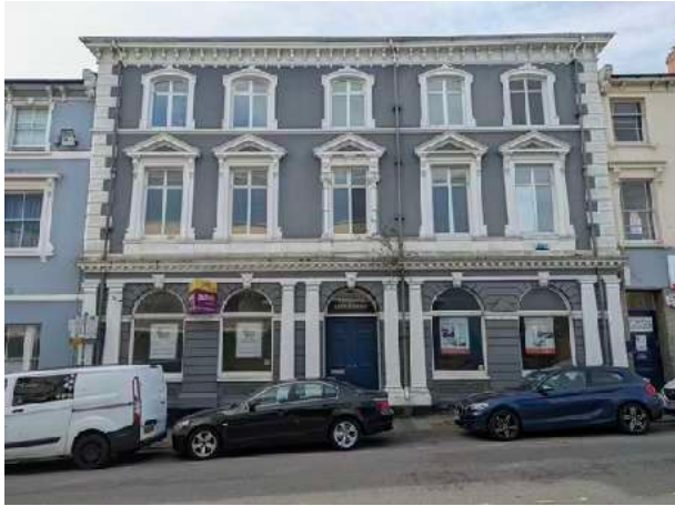
1. Regency Chambers, 20 Bridge Street
