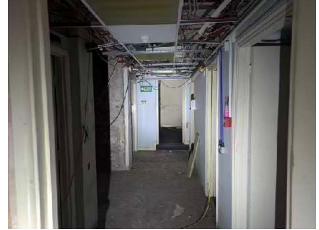
15. Basement circulation space
