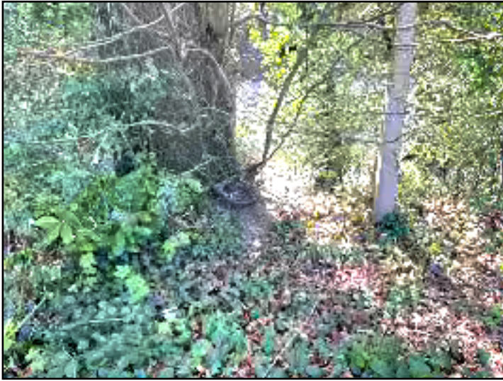
Photo 7. Gap under southern fencing.
