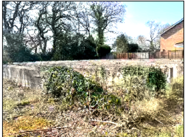
Photo 10. Concrete slabs in centre of site.
