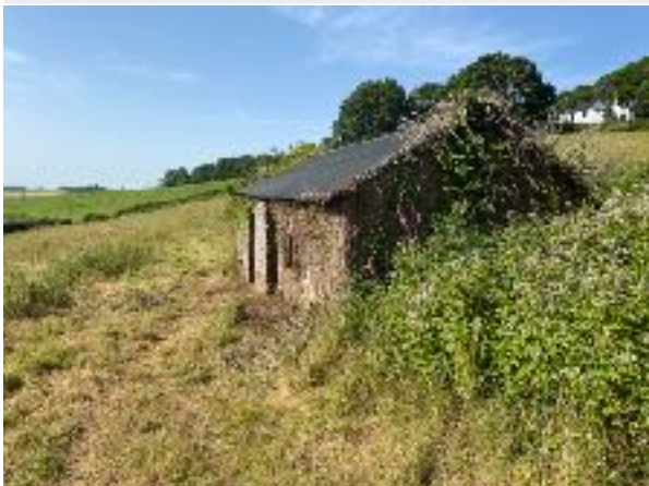
Bramble scrub adjacent to dilapidated stone cottage - facing south-west
