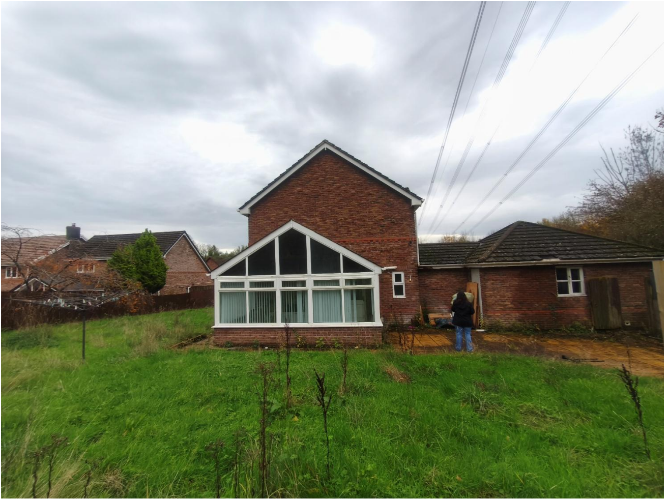
Picture 1: View of rear elevation (from Applicant's rear garden)
