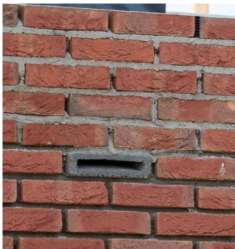
Segovia Woodstone Build-in Bat Box – can be built into wall with entrance only showing at level of finish / surrounding external cladding
