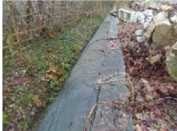
Culverted stream looking west
