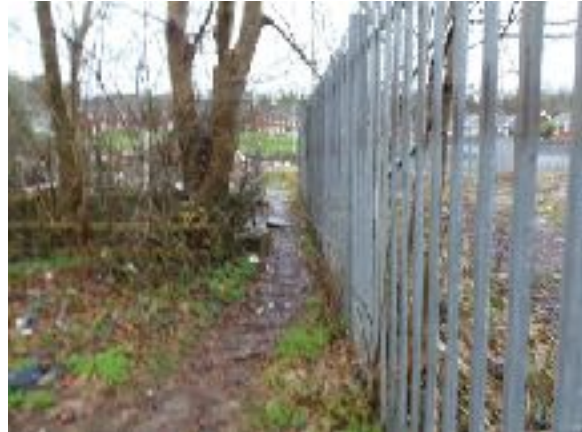
Pathway over culverted stream
