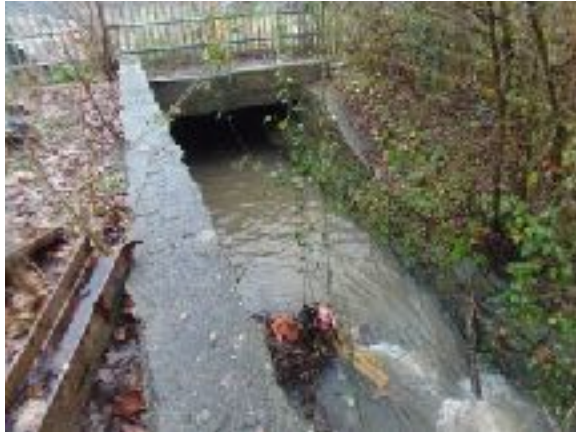
Culverted stream looking east, flowing underneath the concrete hardstanding area
