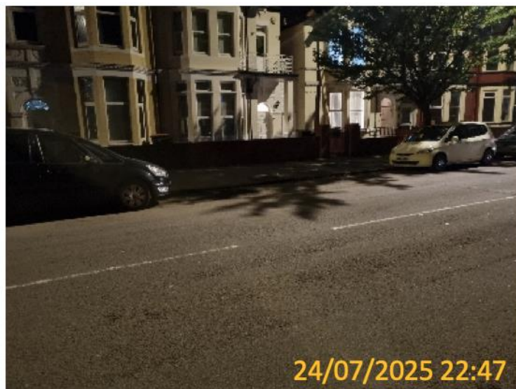
Corporation Road – North Side
