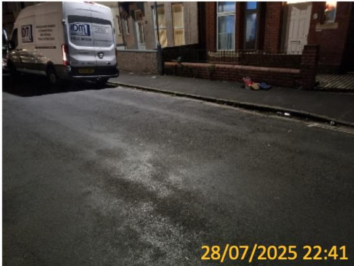
Bedford Road – North Side
